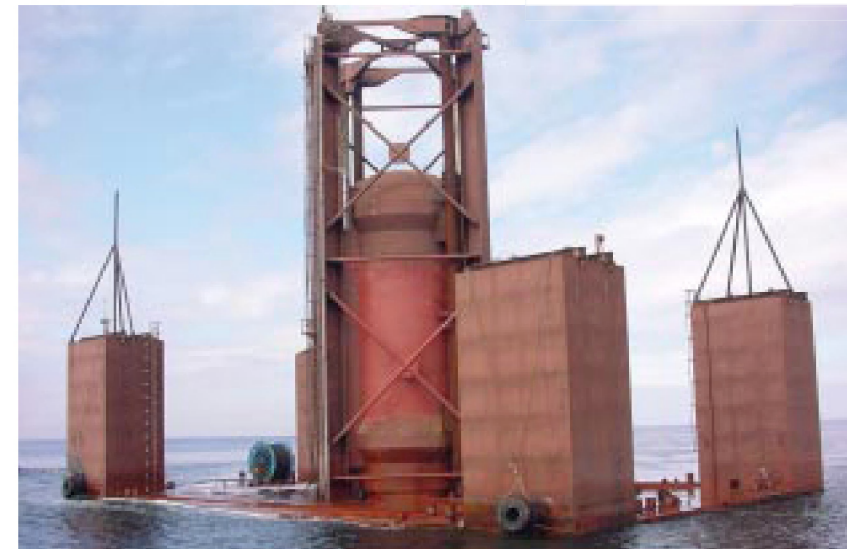
Archimedes Wave Swing Prototype towed to be installed offshore Portugal
