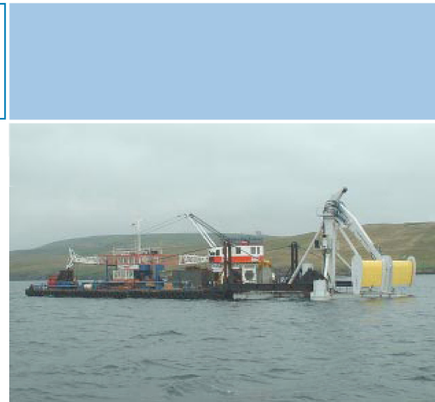
"Stingray" tidal current system in Yell Sound off the Shetland Islands (Courtesy of The Engineering Business, Ltd.)
