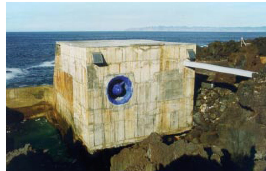
Pico Power Plant at Azores, Portugal
