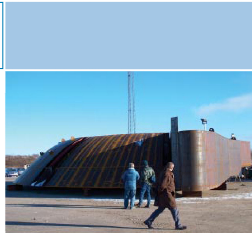
Steel construction of the Prototype Wave Dragon ready for deployment (Courtesy of SPOK)
