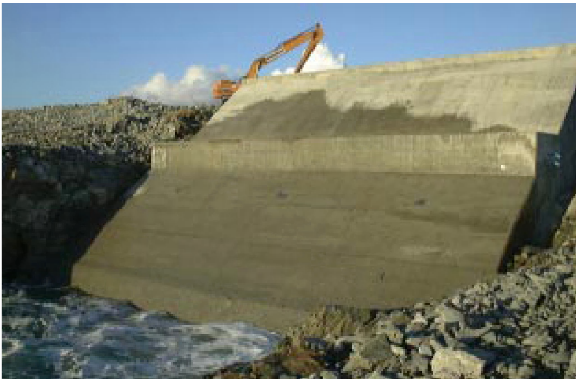
LIMPET power plant at Islay, Scotland (Courtesy of Wavegen)
