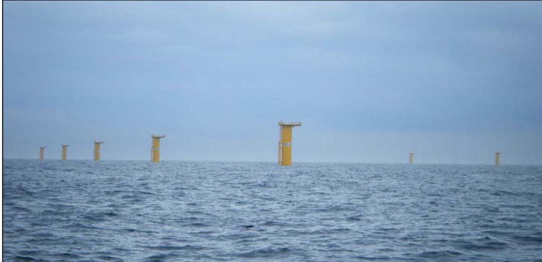
Figure 11. Installed MPs with transition pieces (yellow) on the Bligh Bank (Photo RBINS).
