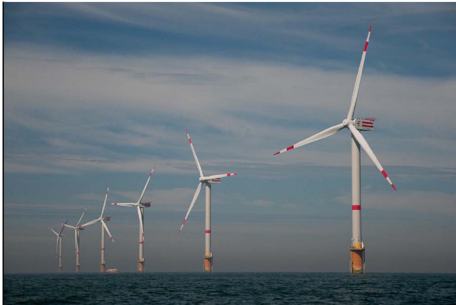
Figure 6. C-Power phase-I on the Thorntonbank produces electricity since May 2009 (Photo RBINS).
