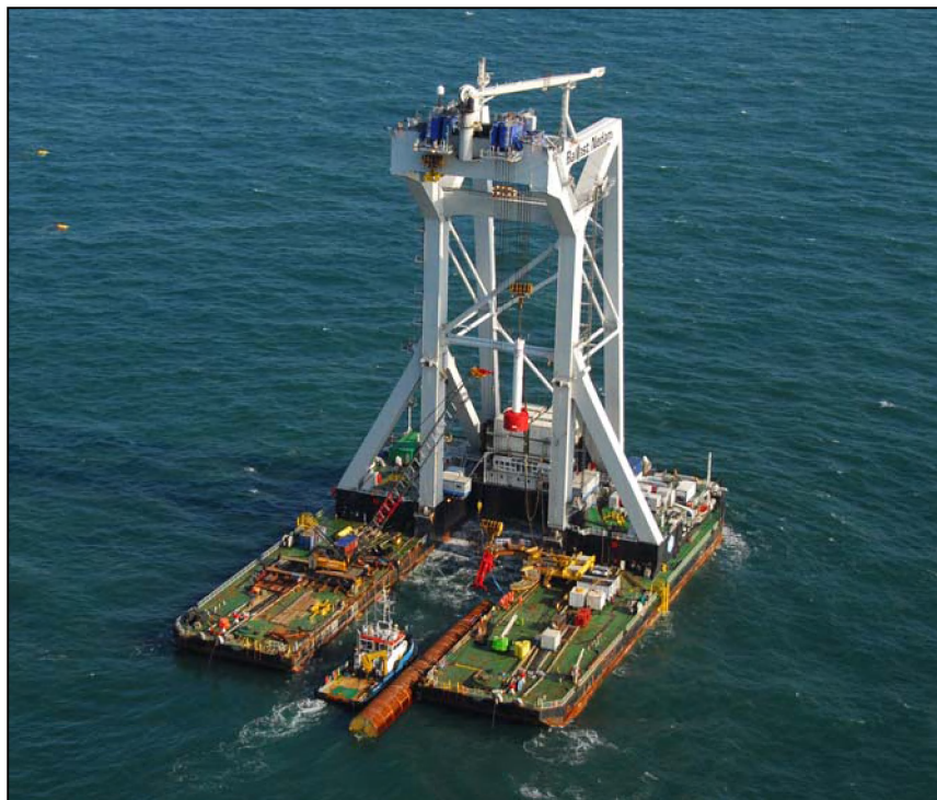
Figure 8. The piling vessel Svanen, with a monopile ready to be lifted and piled and the red and white hammer central in the image (Photo RBINS).
