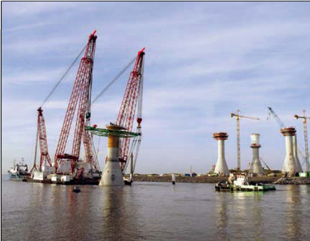
Figure 3. Transport of a GBF from the port of Ostend to the Thorntonbank (Peire et al. , 2009)
