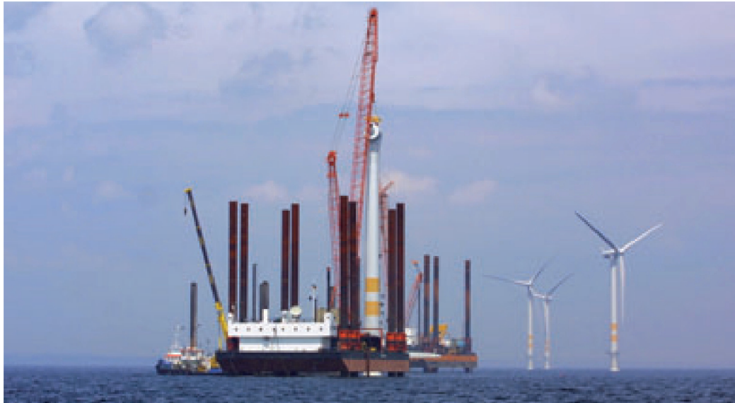
Construction of Utgrunden Wind Farm in Sweden. Photo: Gunnar Britse
