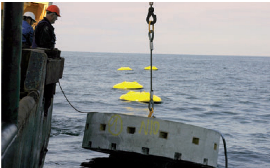
Figure A3-7: Deployment of a wave energy foundation that has been perforated with holes to investigate how it may enhance abundance of fish and crustaceans (Langhamer & Wilhelmsson, 2009). Photo: O. Langhamer.
