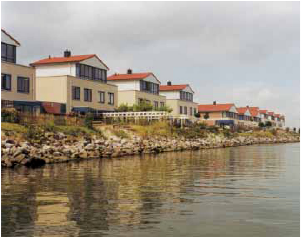
Construction of housing units on the outside of the dike along the IJsselmeer (Photo: RWS-Directorate IJsselmeer area)
