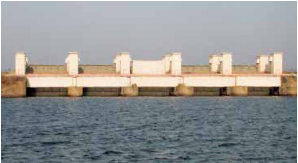
The locks in the Afsluit dike sluice by gravity (Photo: RWS-Directorate IJsselmeer area)
