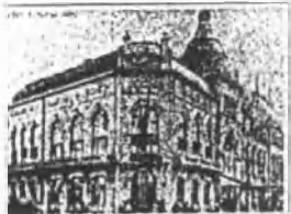
Théâtre royal ('Casino'), Oostende Architect Chambon
