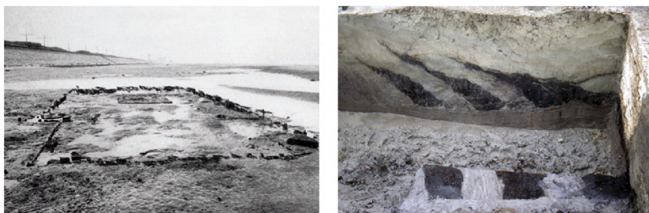
FIG. 5 Left: Ground-plan of a late medieval house on the beach of Raversijde (After Chocqueel 1950). Right: Excavation of the Roman dyke in Walraversijde. The dyke is made up of carefully stacked clay blocks. Wedge-like peat sods (dark colour) were used to reinforce the western side of the dyke, in the forefront a horizontal cross-section of the same peat sods. The latter clearly indicate three successive reinforcement phases of the dyke.
