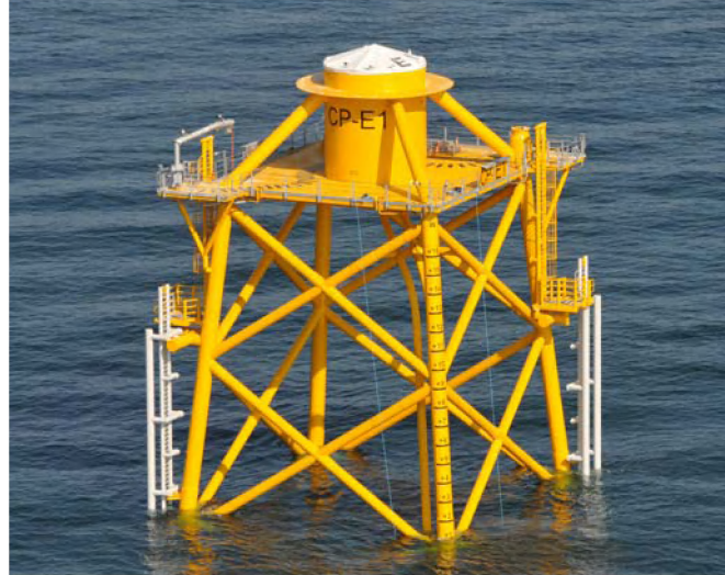
Figure 3. Photo of a jacket foundation of C-Power (Photo RBINS / MUMM).
