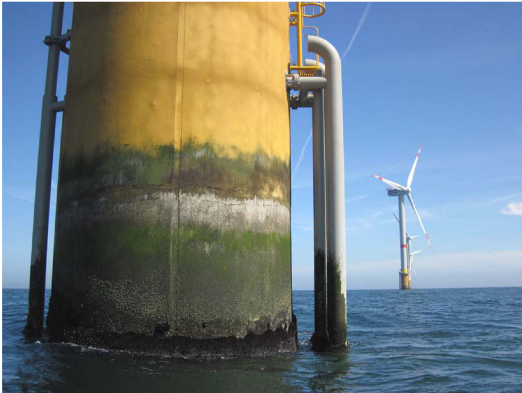
Figure 1. Concrete C-Power GBF foundation (D5) with epifouling in the eulitoral and splash zone (situation early 2011).
