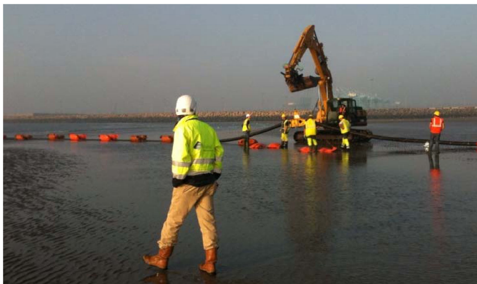
Figure 7. Preparation of the beach pull in of the export cable at Zeebrugge (Photo Belwind).
