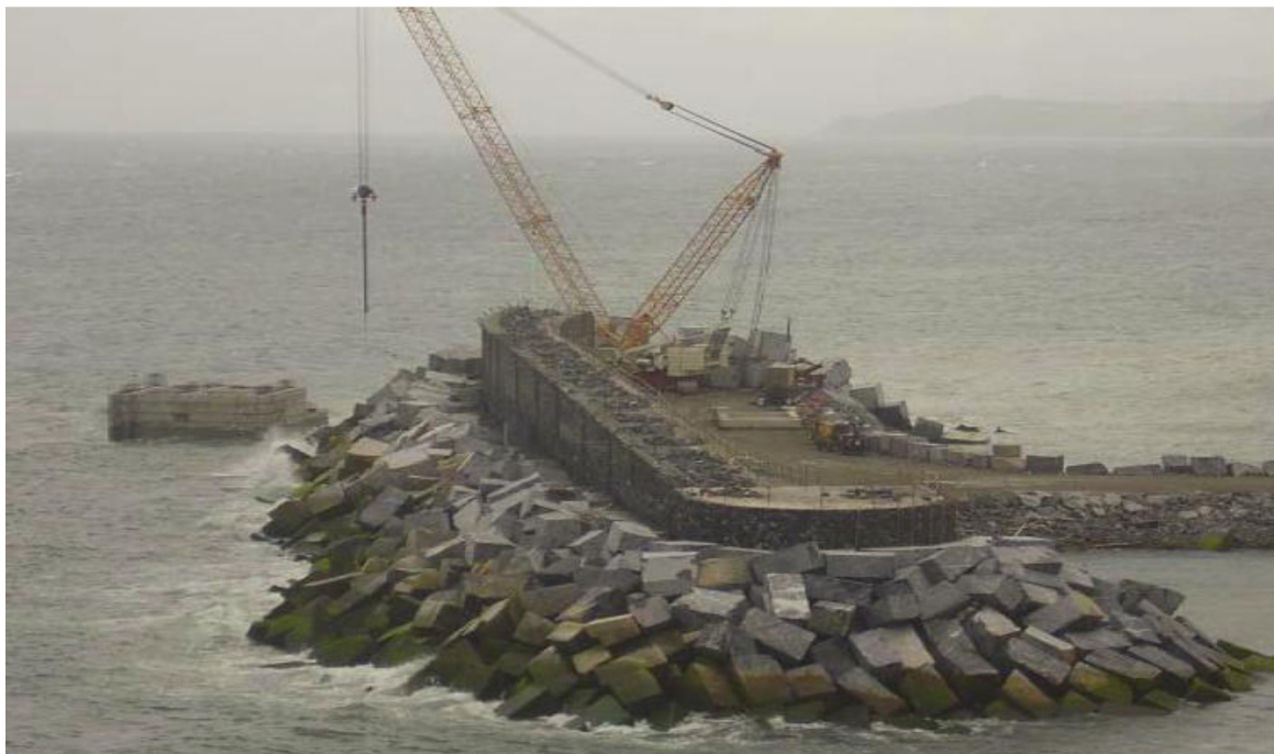
Figure 10: Construction of the Mutriku breakwater and air compression chambers (left).
