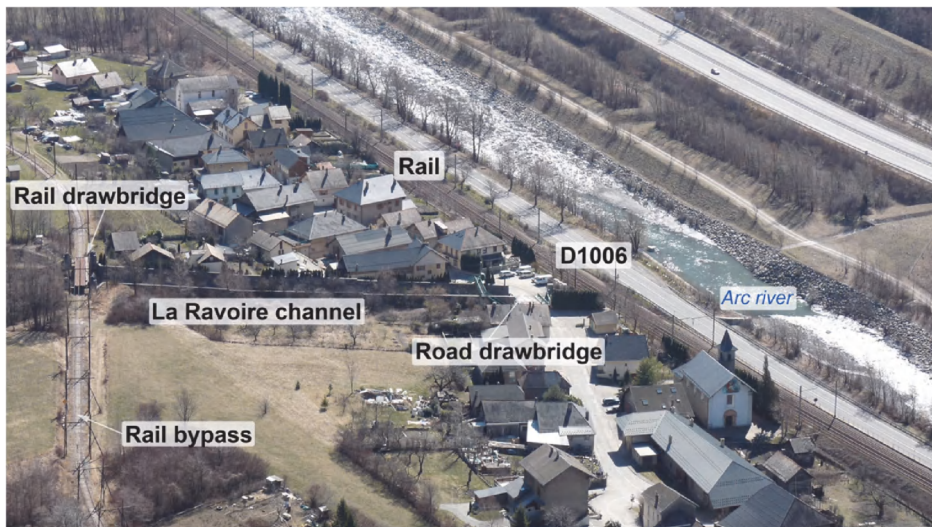
Fig. 8. View of Pontamafrey village constructed on the debris cone of La Ravoire. La Ravoire channel crosses the village the international line of high-speed train (TGV) which links Paris to Turin and the road way D1006.
