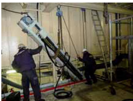
Placing the Hipap cylinder, to get it in was quite an achievement.
