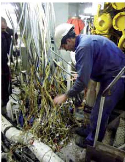
Sorting out the wires for the new Alarm and Monitoring System.
