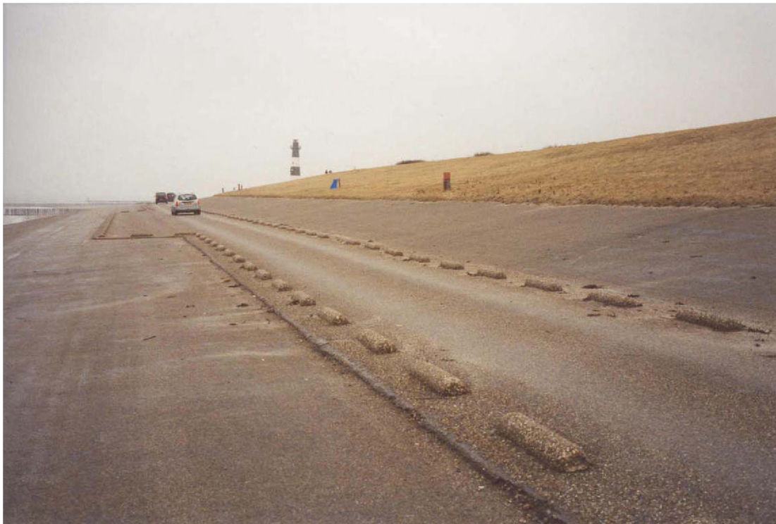
Asphalt revetment on the seaward side of the dike.
