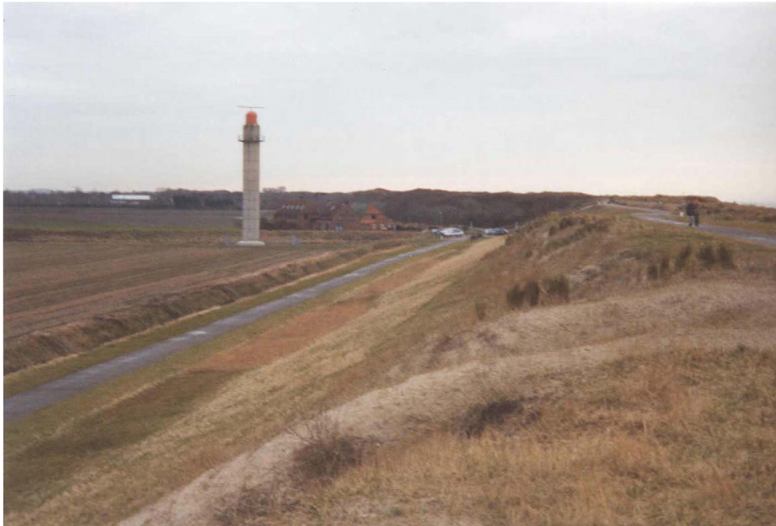
The landward side of the dike primarily has a grass cover.
