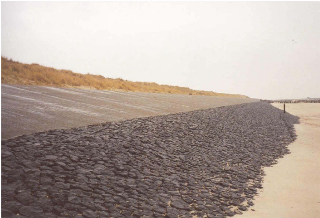
Stone pitching, asphalt revetment on the seaward side of the dike.
