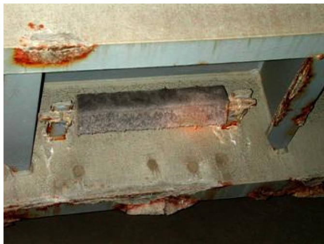
Figure 110: A poorly sited anode (Amtec, 2008)
