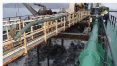
Figure 2. Dredging sand and gravel from the seabed in Kollafjörður.
