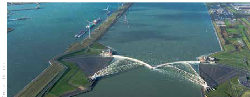
The Maeslantkering is a storm surge barrier in the Netherlands, which automatically closes when needed for protection.
