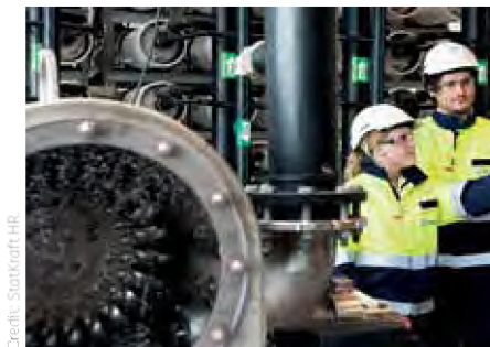
In an osmotic power plant, the pressure created from the membranes is utilised through a turbine to generate electricity.
