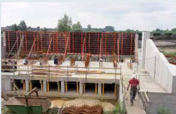
Figure 7.9. Formwork and reinforcement of the superstructure
