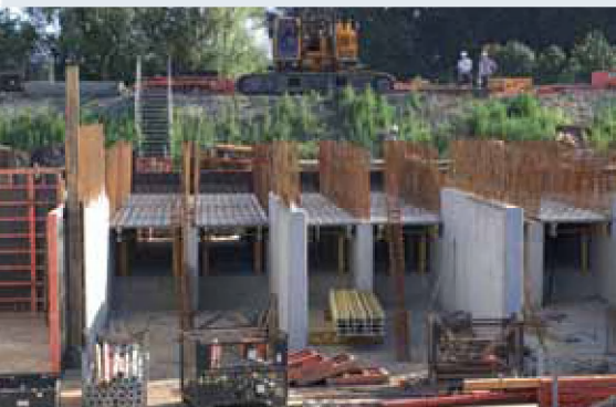
Figure 7.8. Formwork and reinforcement of the intermediate plate of the inlet and outlet
