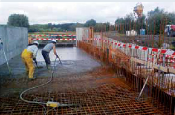
Figure 7.6. Floor slab and sheet piles against seepage
