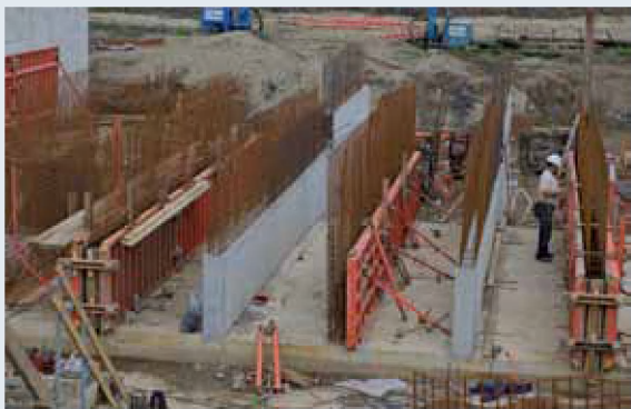
Figure 7.7. Concreting the walls
