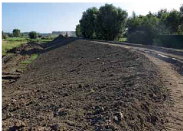
Figure 7.2. Earthworks: raising and widening the ring dyke
