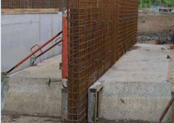
Figure 7.5. Formwork and reinforcement of the walls
