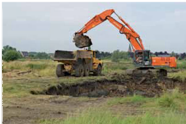
Figure 7.1. Earthworks: start of excavating the channel source
