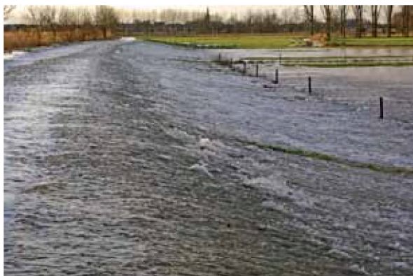
Figure 1.4. Scheldt water flooding over the overflow dyke in the Paardeweide FCA
