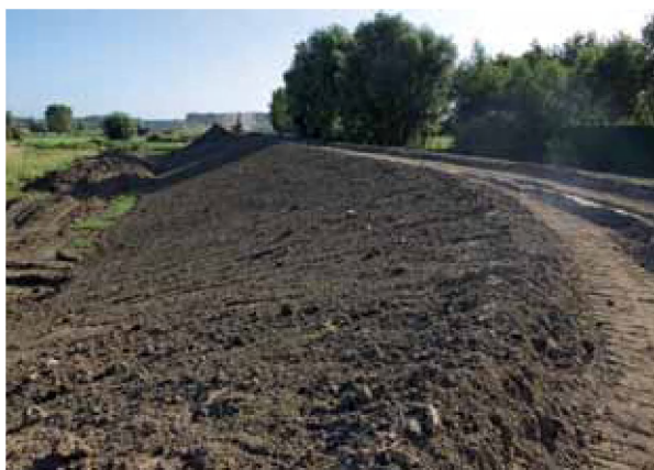
Figure 7.2. Earthworks: raising and widening the ring dyke
