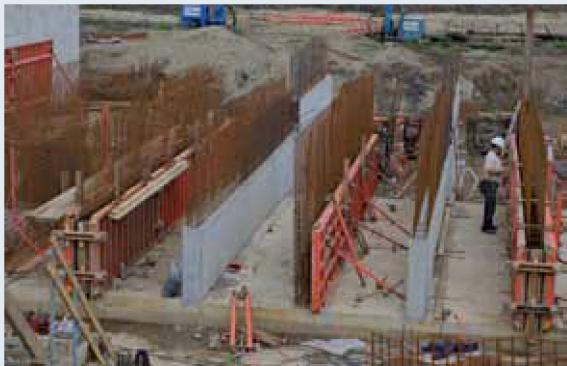
Figure 7.7. Concreting the walls
