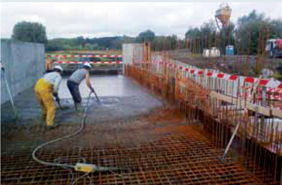
Figure 7.6. Floor slab and sheet piles against seepage
