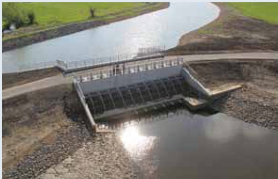
Figure 7.11. Finished sluice
