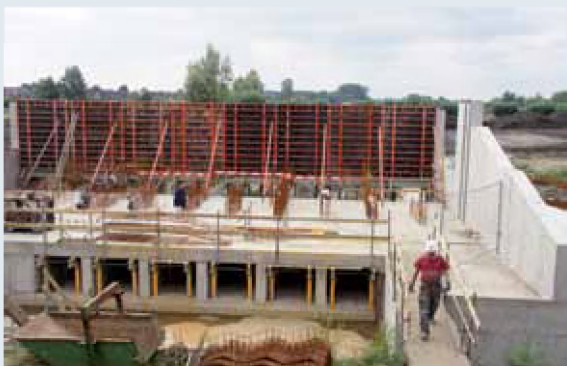
Figure 7.9. Formwork and reinforcement of the superstructure
