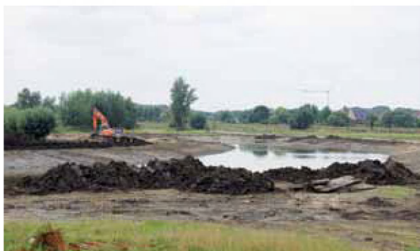
Figure 7.3. Earthworks: end of excavating the channel source
