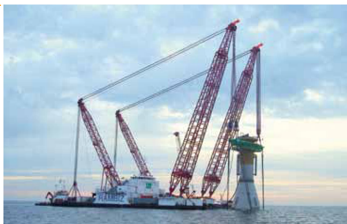
Transport of a gravity based foundation from the port of Ostend to the C-Power site at the Thorntonbank.
