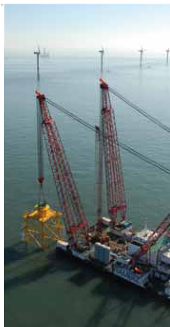
Phase 3 jacket installation at the C-Power site.
