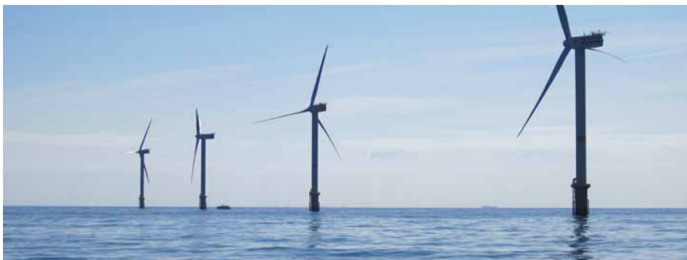
Turbines with gravity based foundations on the Thorntonbank.
