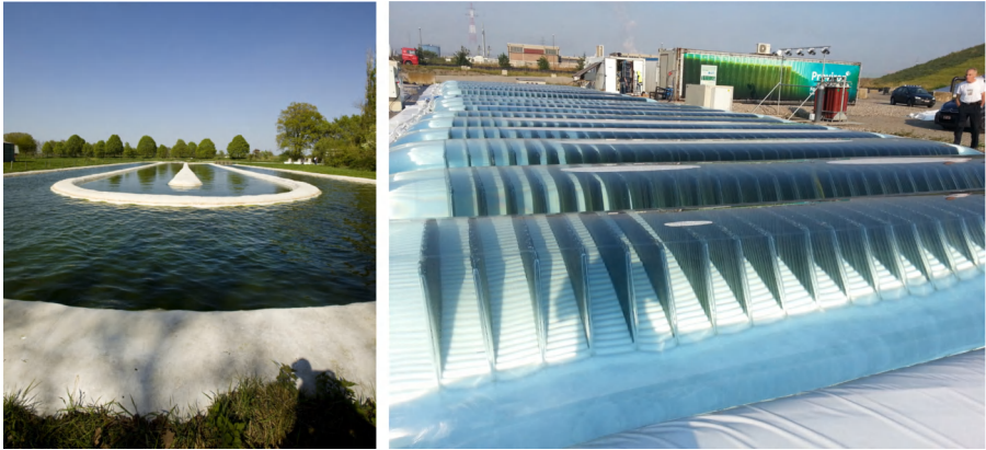
Figure 1.3: Example of open raceway pond reactors (Ingrepo, The Netherlands) and a novel design of a low-cost photobioreactor (Proviron, Belgium) [187].
