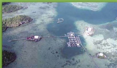
Igang Marine Substation
