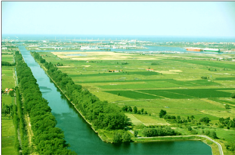
Figure 3.5. Aerial photograph of the development area ( http://www.ministerhildecrevits.be/ ).
