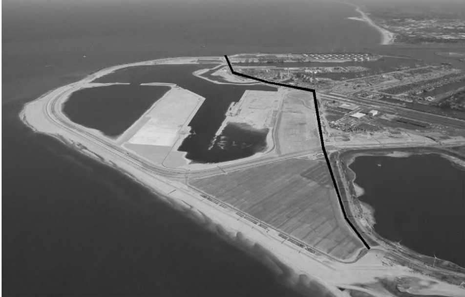
Figure 8 Aerial view in July 2012 of the genesis of Maasvlakte 2 (left from black line). The line indicates the border between Maasvlakte 1 (right) and Maasvlakte 2 (left)(see Fig. 1). Photograph by Aeroview, Rotterdam, the Netherlands.
