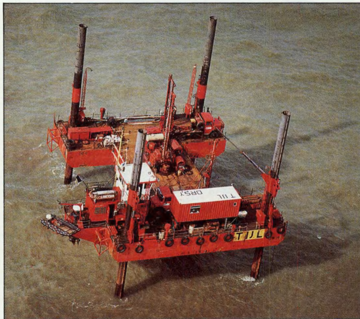
The self-propelled jack-up platform "Tijl" was employed during compaction works carried out by explosives; equipped with three jetting rigs, the platform was moved in parallel lines to minimise anchor movements.
