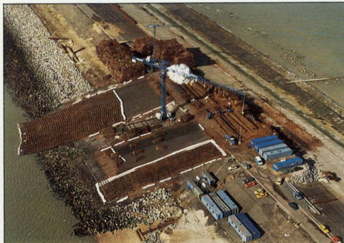
Manufacturing in progress for the willow mattresses, provided for protection against erosion and scour of both sides of breakwaters.
