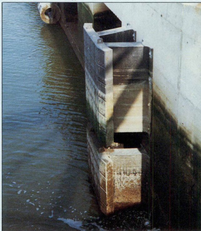
A series of fenders was supplied by Sumitomo Rubber Industries Ltd. of Japan through their Brussels office for the new sea lock. This lock was built by a joint venture of SBBM Enterprises and SOGETRA to provide access for ships of up to 125,000 d.w.t. to the new docks in the inner harbour. Photo shows Pi-type 1250 H x 2750 L fender.
