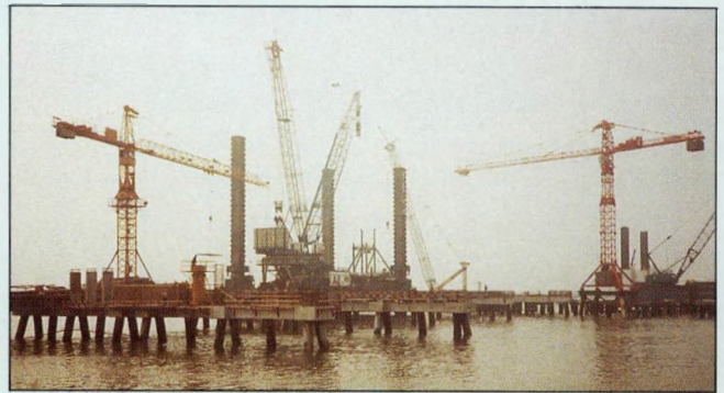
Begemac N.V. of Antwerp supplied longitudinally welded steel pilings with an outside diameter of 914.3 \times 14\text{ mm} wall thickness and in different lengths of between 25,050 and 28,790 mm for the LNG terminal (as shown in the photo). The company also supplied longitudinally welded tubular steel dolphins with a diameter of 2,200 mm and in different wall thicknesses of between 25 and 58 mm.
