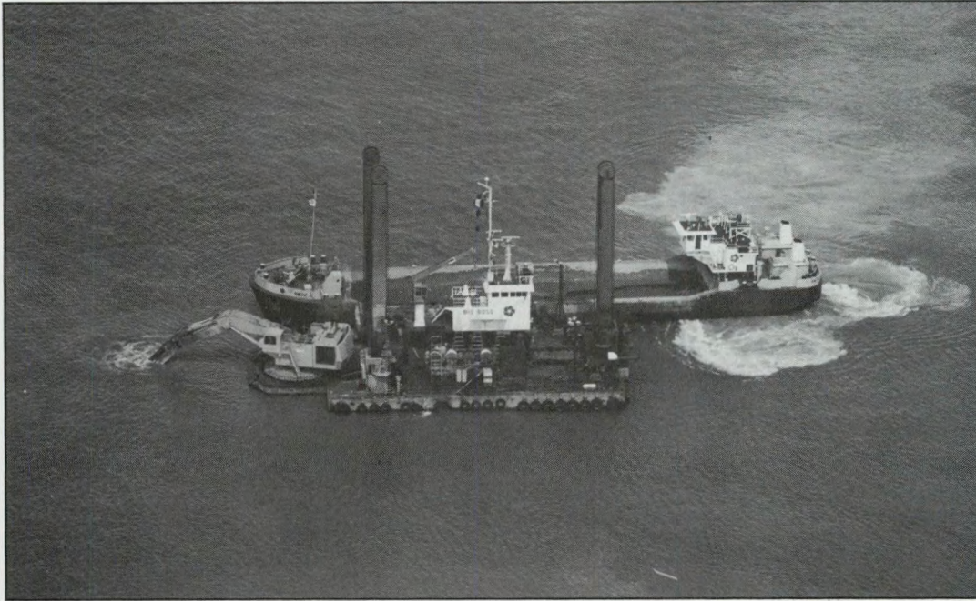
Soils that could not be used for reclamation were loaded by Dredging International's backhoe dredger "Big Boss" into 1,000 m 3 split hopper barges.
