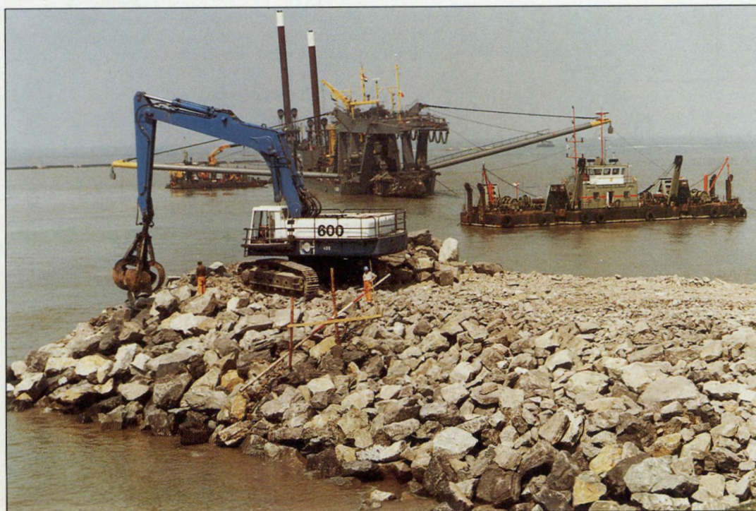
Construction of the front of the eastern breakwater, with dredging of unsuitable topsoil being undertaken by the "Oranje".
