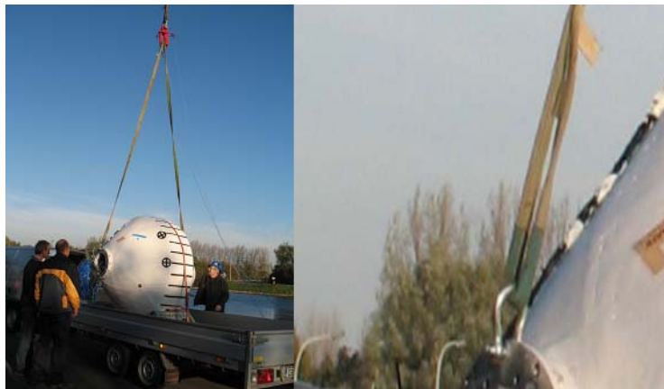
Figure 9-55 Two elastic cables used to lift the buoy (left) and detailed picture of elastic cable to a lifting eye bolt (right).
