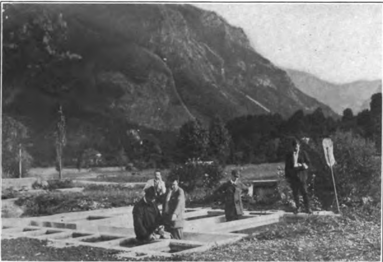
B. OUT-OF-DOOR CEMENT CULTURE BASINS.
