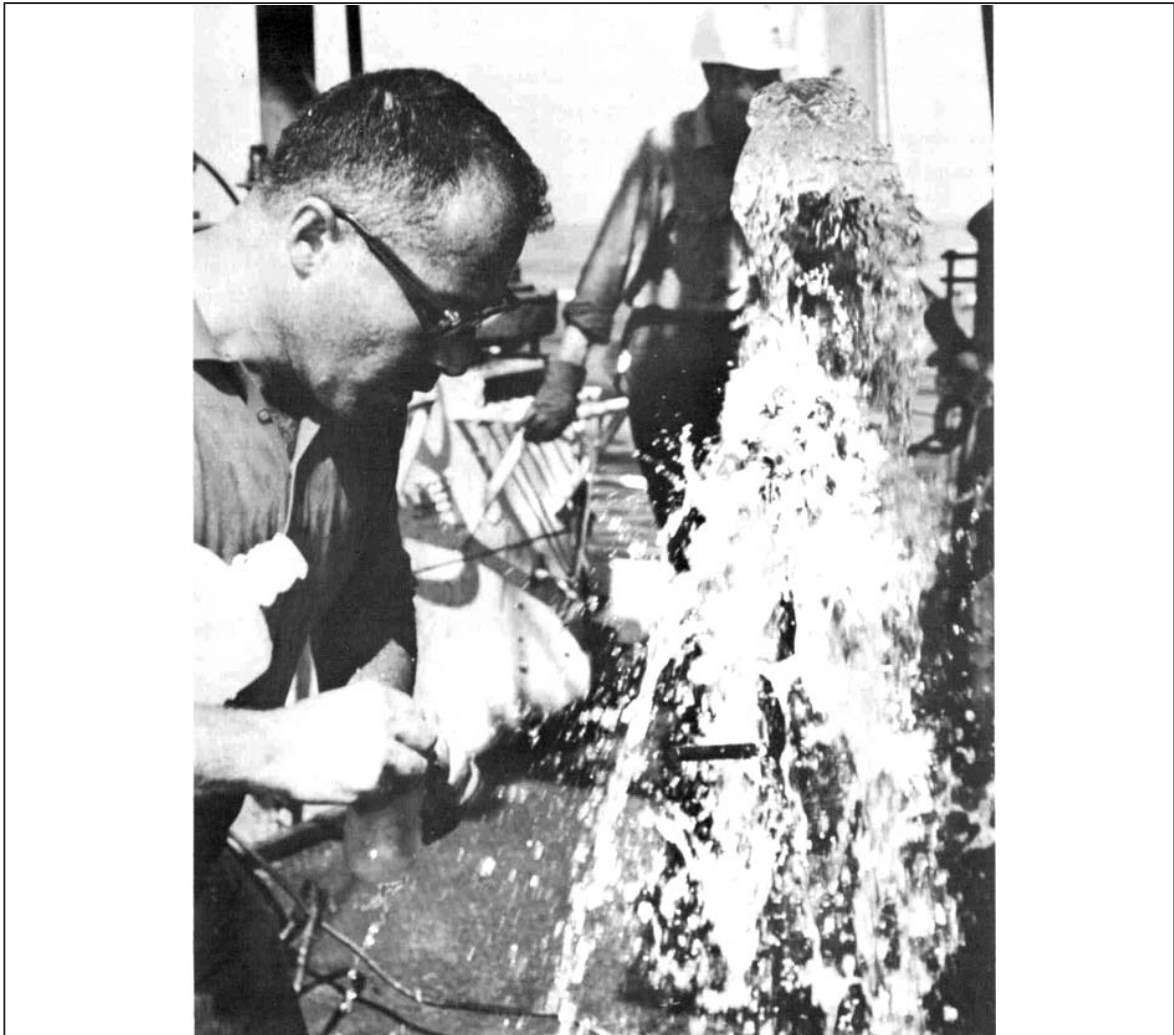
Figure 3. Well J1A, a geologic exploratory well 43 km offshore from Jacksonville, Florida penetrated an artesian aquifer that flowed up the drill pipe. The water, with a chloride content of only ~700 ppm (seawater = 19,000 ppm Cl), came from a depth of 250 m below the ship and had a hydrostatic head of 9 m above sea level.
