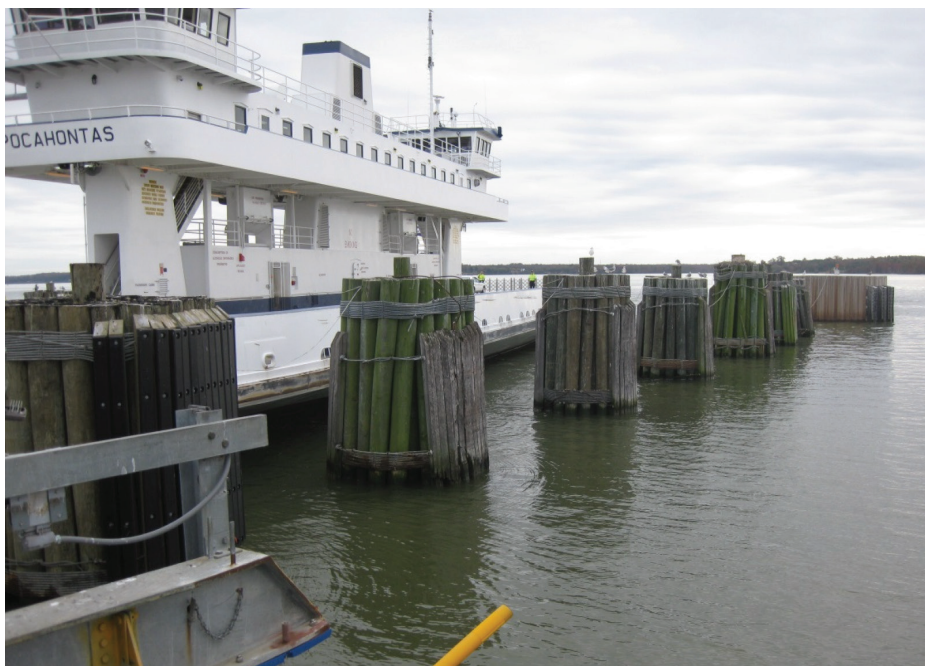
Figure 3: Typical dolphin arrangement (Courtesy of VDOT)
