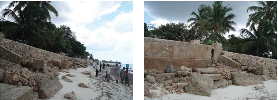
Fig. 47. Failing seawalls with block aprons between Kawe and the Mbezi River, Kunduchi shore. Photos Y.W. Shaghude.
