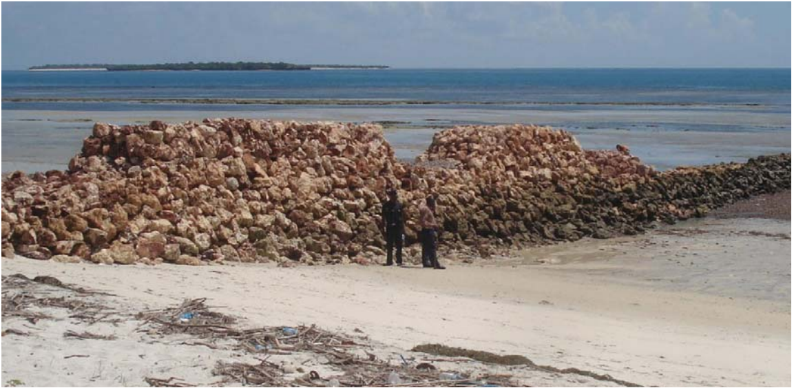
Fig. 48. Groyne constructed of quarried rock blocks on the Kunduchi shore between the Beachcomber and Whitesands hotels (see Fig. 49). Photo Y.W. Shaghude.
