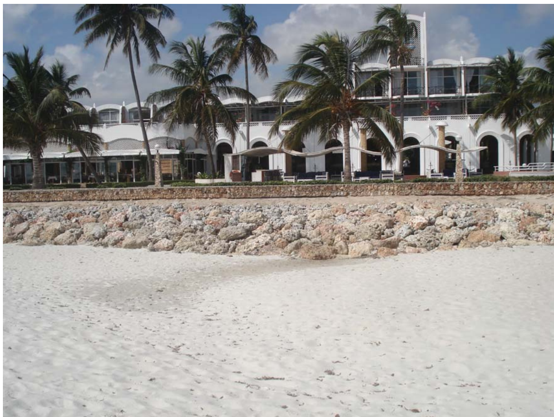
Fig. 36. Seafront hotel protected by a rock-block revetment and capping wall, Kunduchi site. Photo: Y.W. Shaghude.
