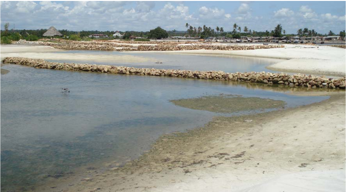
Fig. 50. Groynes comprising quarried rock blocks installed on the Kunduchi shore north of the Beachcomber Hotel, at the site of the former Africana Hotel (see Fig. 49). Photo R.S. Arthurton.
