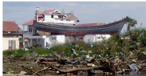
Runup can often be inferred from the vertical extent of dead vegetation, from debris normally found at ground level that are observed stuck on electric wires, in trees, or at other heights, and from water line marks left on building walls. In extreme cases, cars, boats, and other heavy objects have been lifted and deposited atop buildings. Banda Aceh, Indonesia, 26 December 2004. Photo courtesy of C. Courtney, Tetra Tech EMI.
