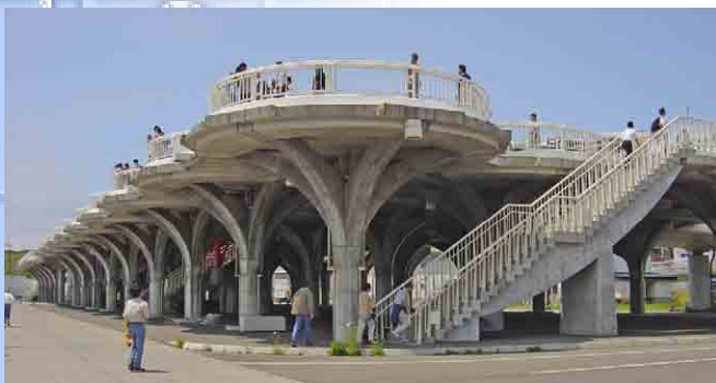
Elevated platform used for tsunami evacuation that also serves as a high-elevation scenic vista point for tourist. Okushiri Island, Japan. Photo courtesy of ITIC.
