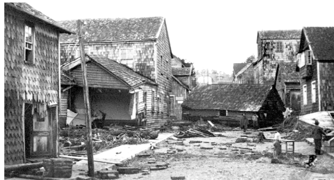
Damaged caused by the 22 May 1960 Chilean tsunami. Photo courtesy of Ilustre Municipalidad de Maulin, USGS Circular 1187.
