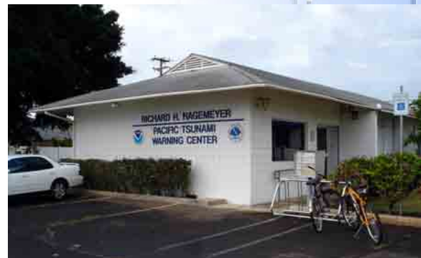
PTWC facilities located at Ewa Beach, Hawaii, USA.
