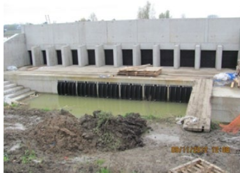
Figure 5 Inlet and outlet sluice configuration in the river side (construction phase) (source: Patrimoniumdatabank W&Z)
