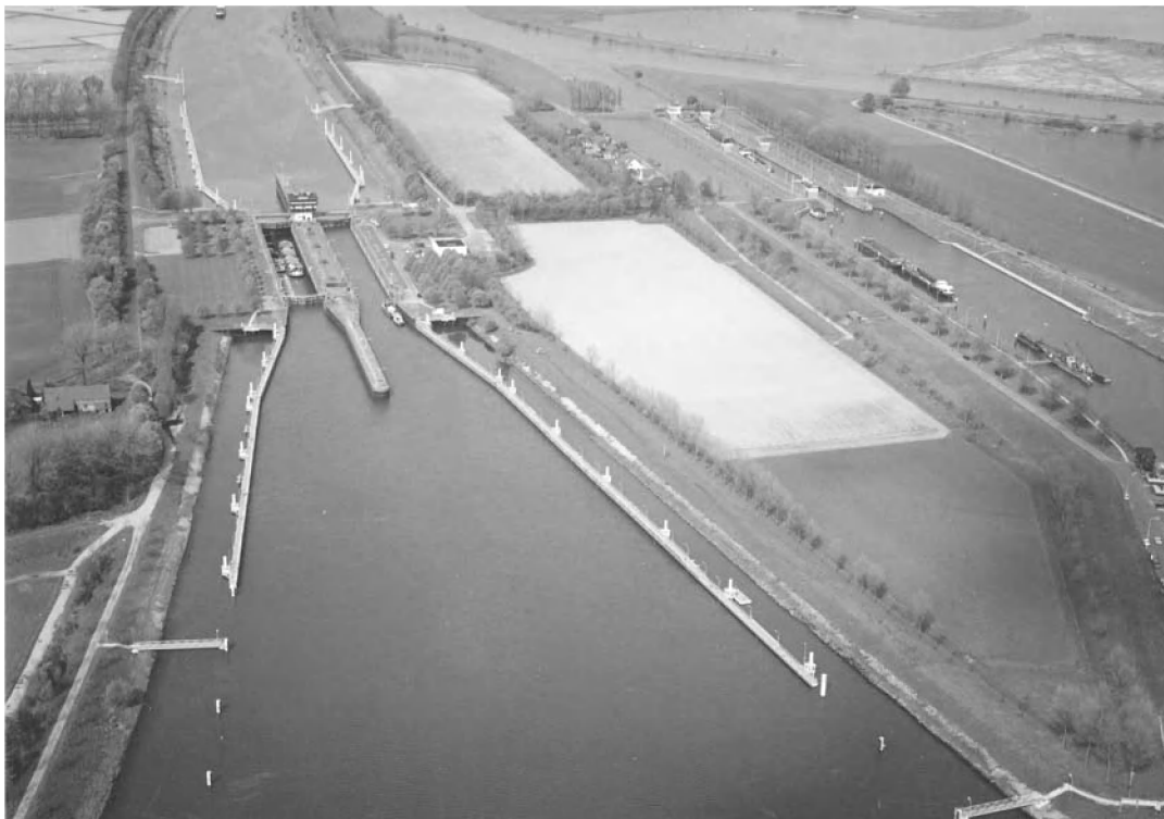
Photo 5.9 Lay out of lock complex in Heel (left) and Linne (right) on the Maas
