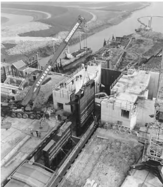
Photo 8.3 Outer head with single pivot gates of the navigation lock at Nieuwe Statenzijl
