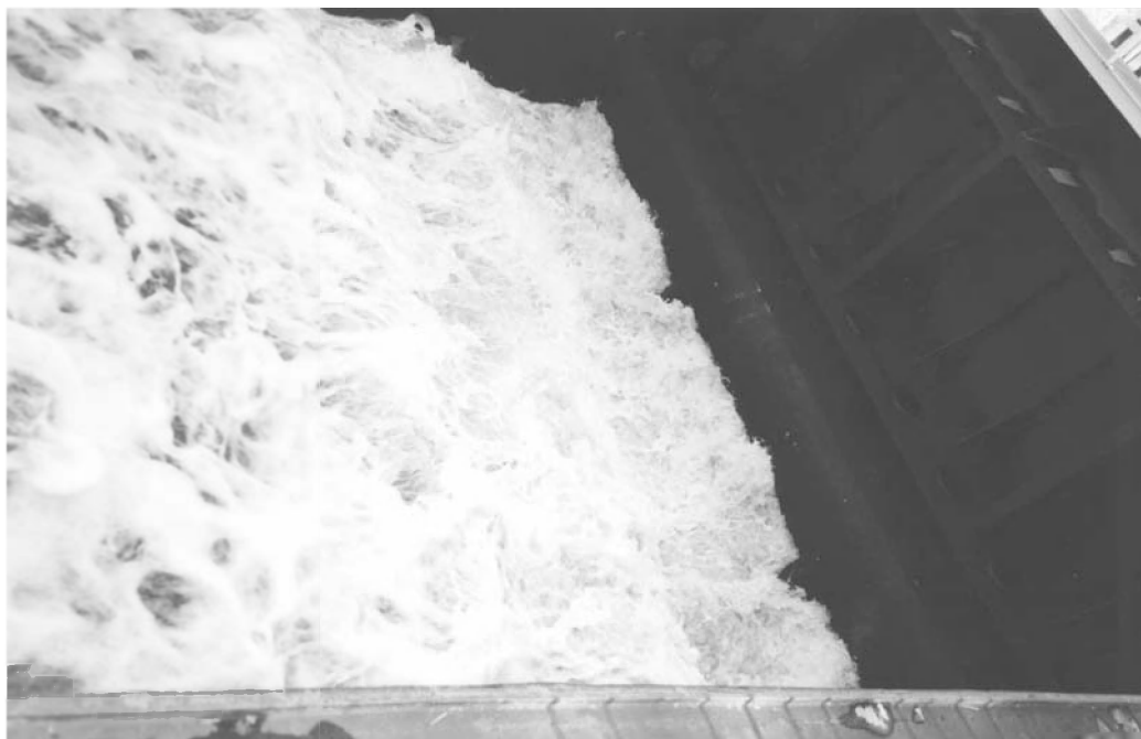
Photo 6.3 Flow pattern during filling by means of lifting the upper gate at the lock in Eefde
