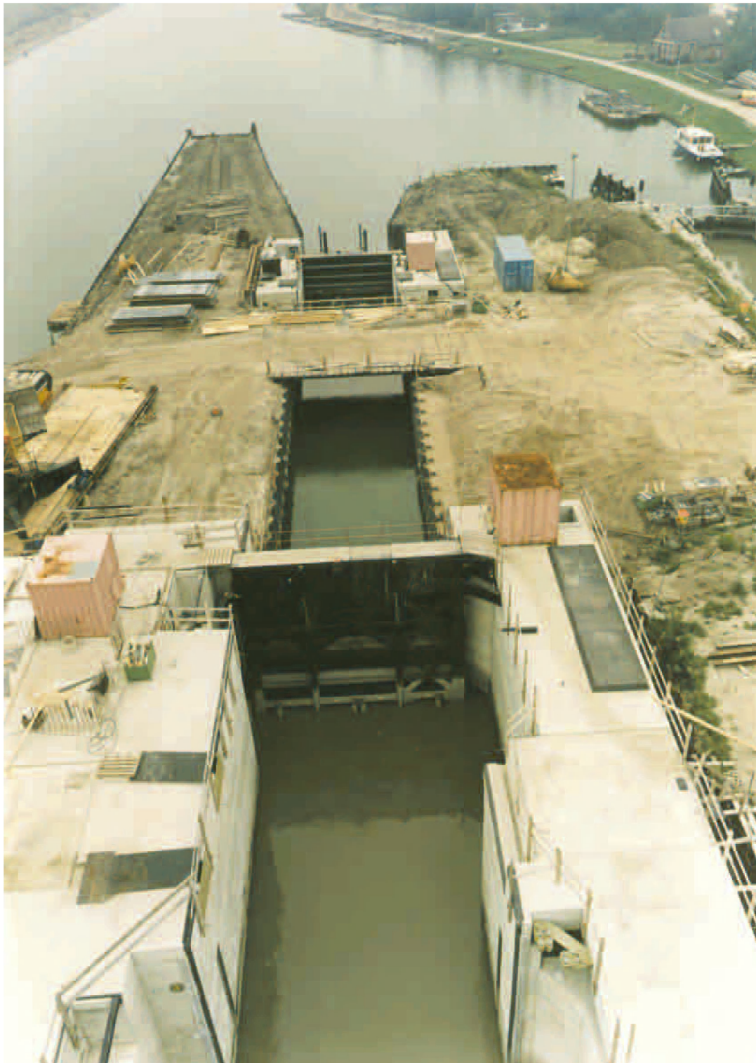
Photo 8.1 Outer head (foreground) and inner head (background) of the navigation lock in Nieuwe Statenzijl
