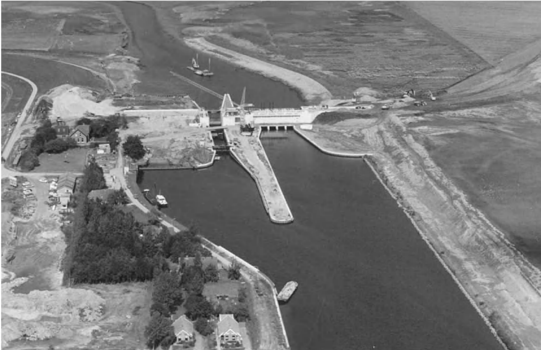
Photo 5.4 Lay out of the lock complex at Nieuwe Statenzijl with navigation lock (left) and drainage lock (right)
