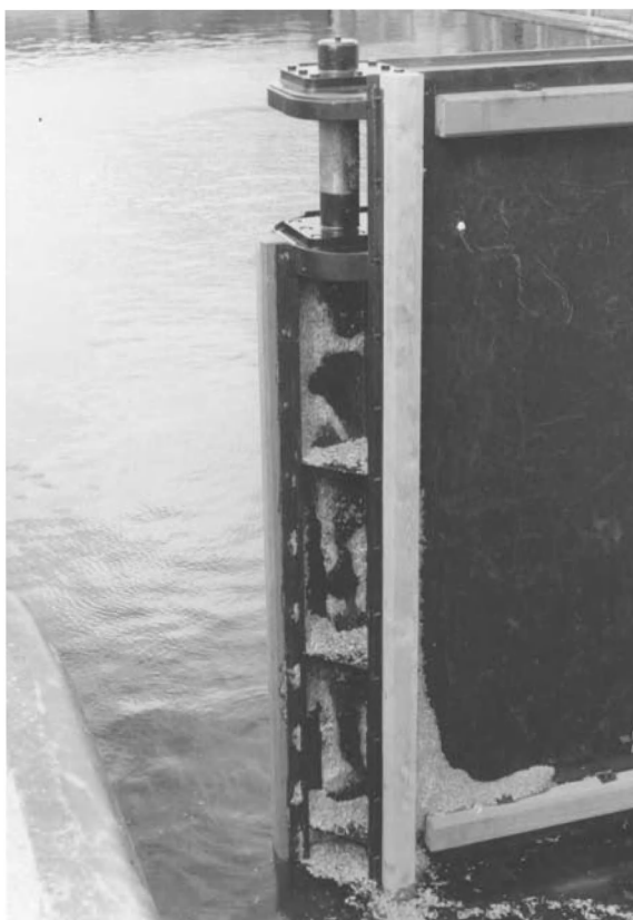
Photo 7.11 Pintle rod of the mitre gate at Middensluis IJmuiden
