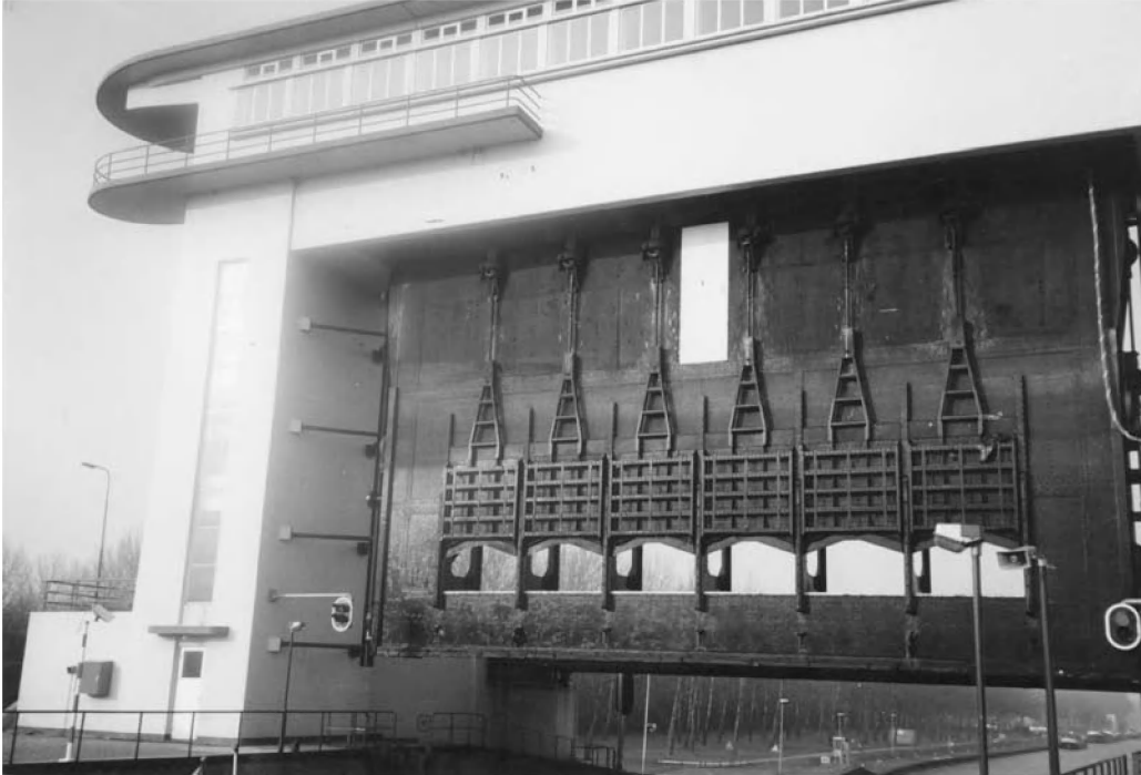
Photo 6.7 Gate openings in the lift gates of the Princess Beatrix locks in Nieuwegein
