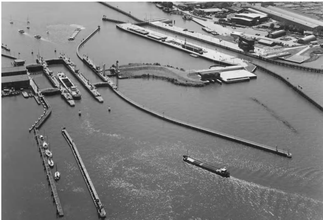
Photo 5.5 Lay out of Oranjesluiscomplex in Amsterdam with (f.l.t.r.) 3 navigation locks, discharge locks and a push-tow lock
