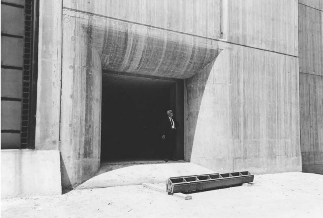
Photo 6.18 Inflow opening of the bypass culvert of the lower head of the locks at Maasbracht
