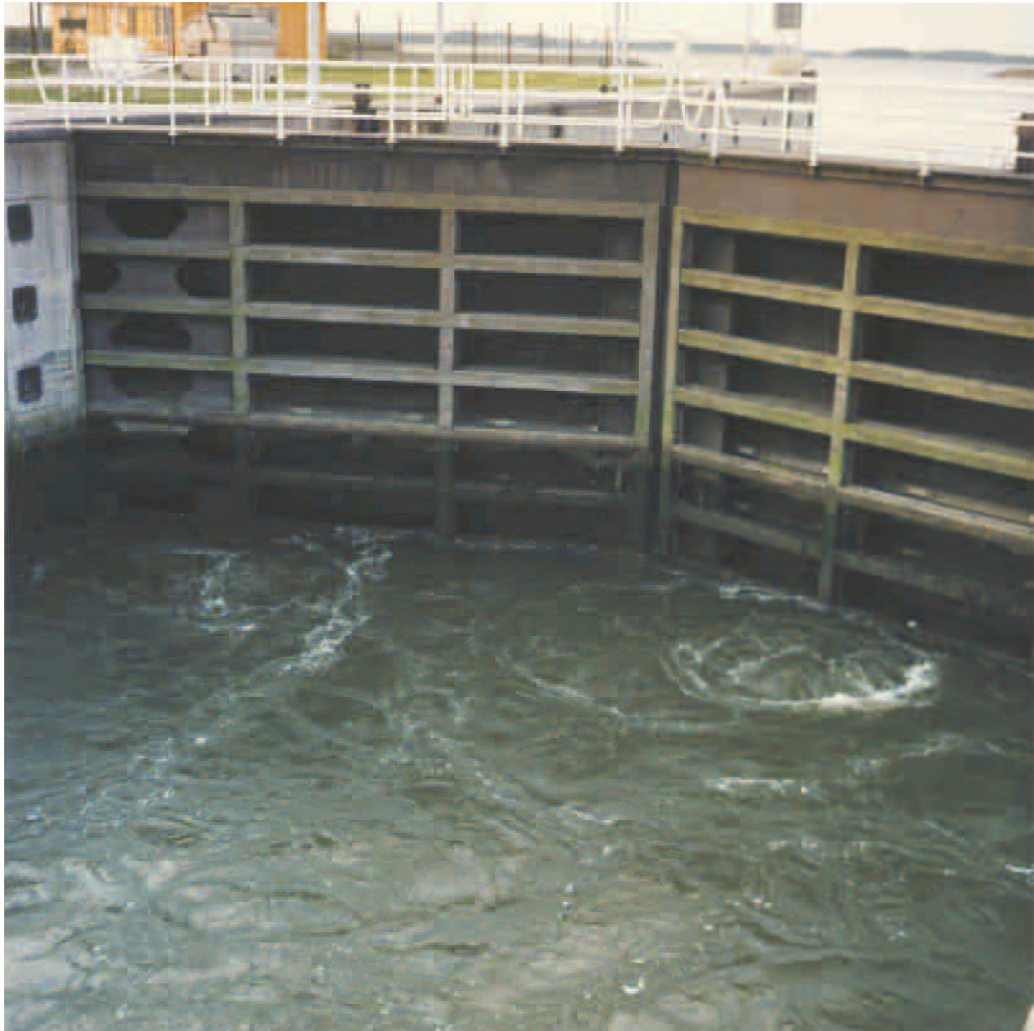
Photo 6.1 Flow pattern during the filling of the yacht lock in the Volkerak
