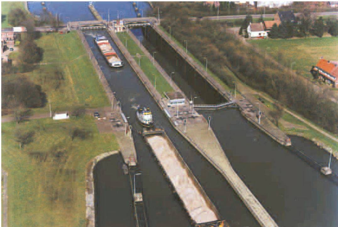
Lock complex Born in the Julianakanaal (March 1999)
