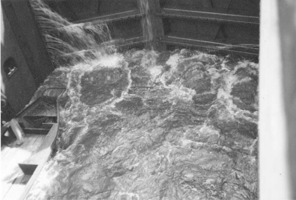
Photo 6.4 Flow pattern during filling by means of gate openings of the lock in the Noord Willemskanaal
