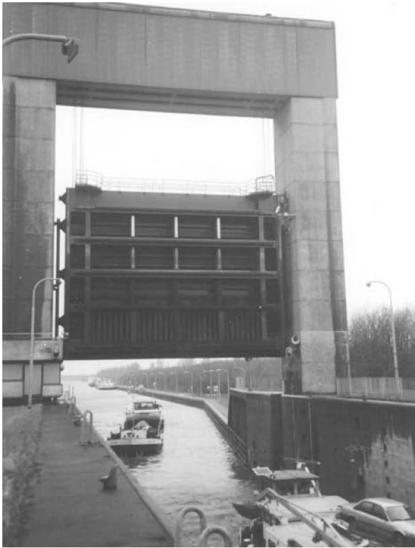
Photo 8.8 Lock head of a lift gate of the new lock in Weurt
