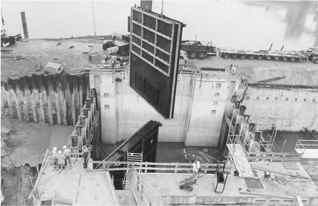
Photo 8.2 Lower head with mitre gates of Tweede Sluis in Lith
