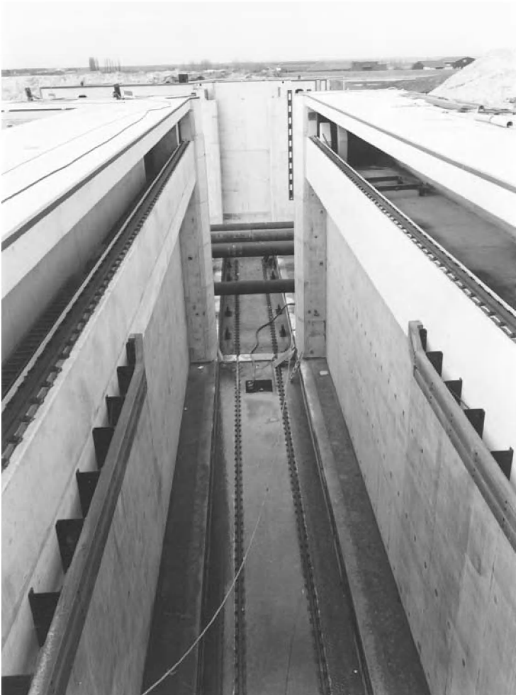
Photo 8.5 Gate chamber of the rolling gate of the push-tow lock in Hansweert
