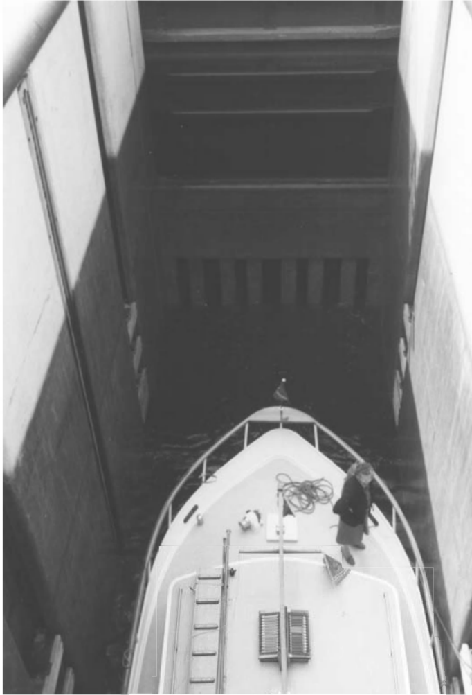
Photo 6.17 Stilling chamber of navigation lock in Almere
