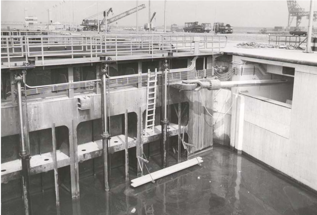
Photo 7.17 Hydraulic cylinder operating mechanism of mitre gates and sluices at Rozenburgse lock
