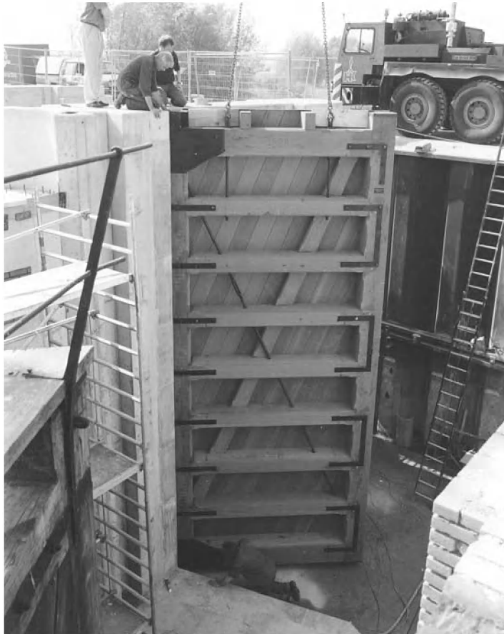
Photo 7.2 Wooden mitre gate of lock at Dalem during positioning (1998)
