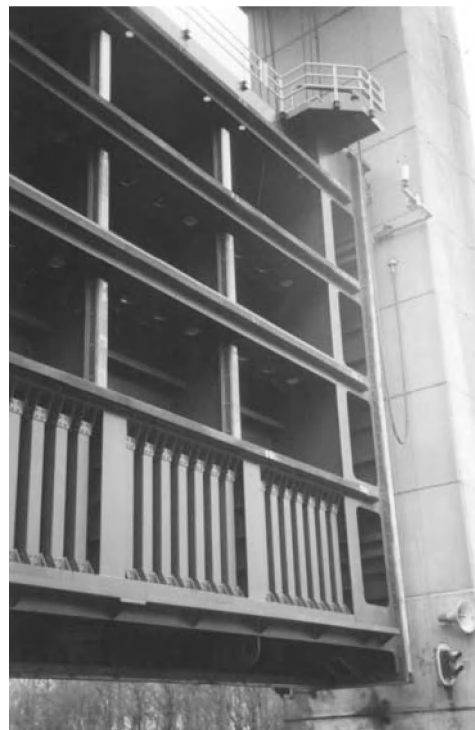
Photo 6.9 Energy dissipating bars behind the rectangular openings in the lift gates of the new locks in Weurt
