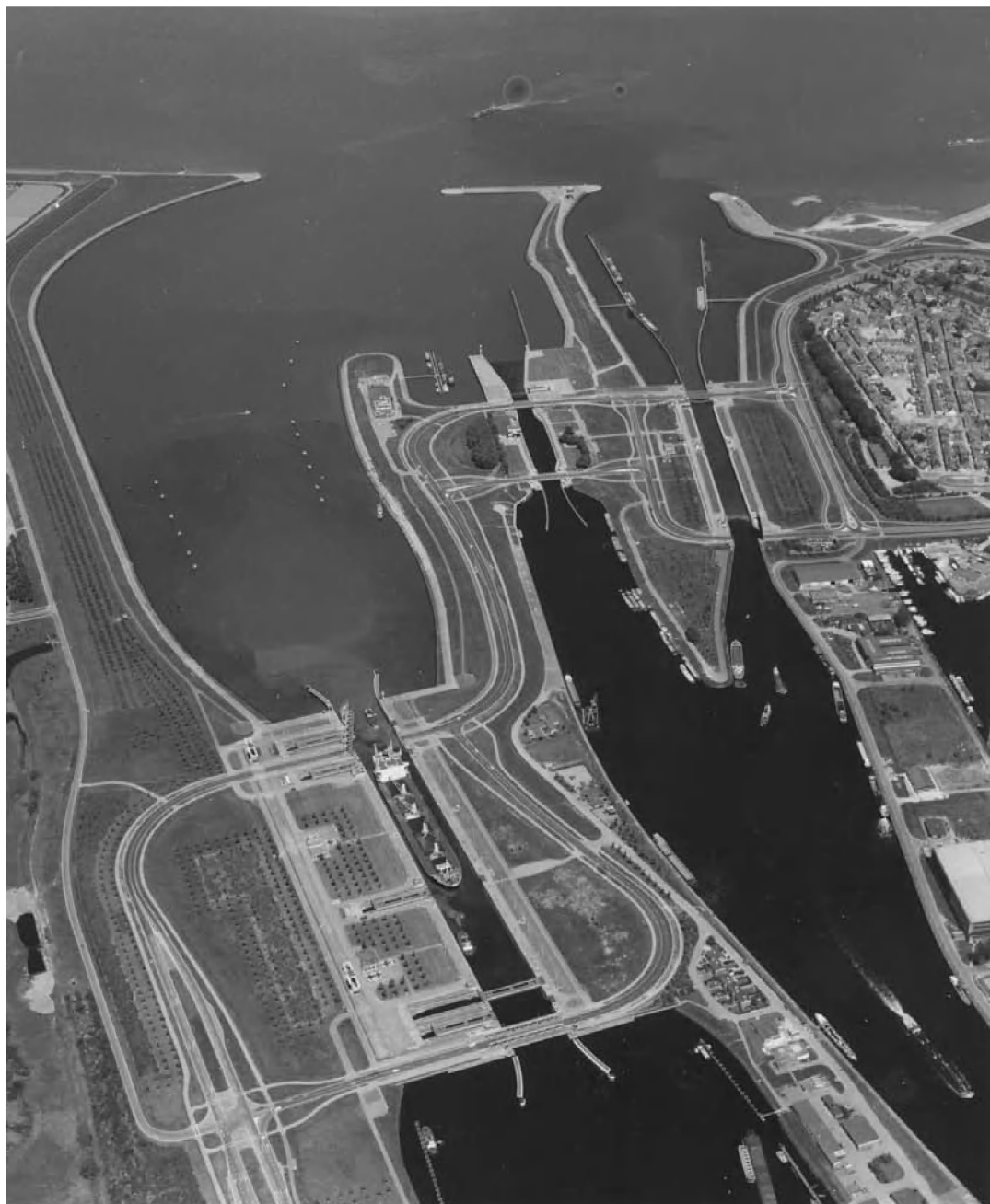
Photo 5.1 Lay out of the lock complex at Terneuzen with (f.l.t.r.) large sea lock, Middensluis and inland navigation lock as link between the Westerschelde (above) with Canal from Gent to Terneuzen (below)
