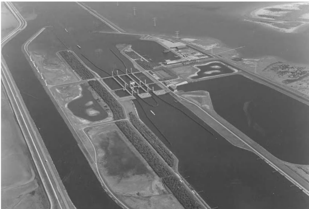
Photo 5.3 Lay out of Kreekraksluizen in the Schelde-Rijnverbinding
