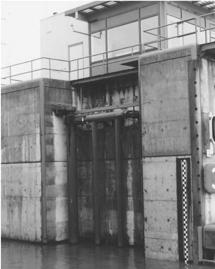
Photo 7.21 Frame shaped locking device for single pivot gate of the lock at Nieuwe Statenzijl
