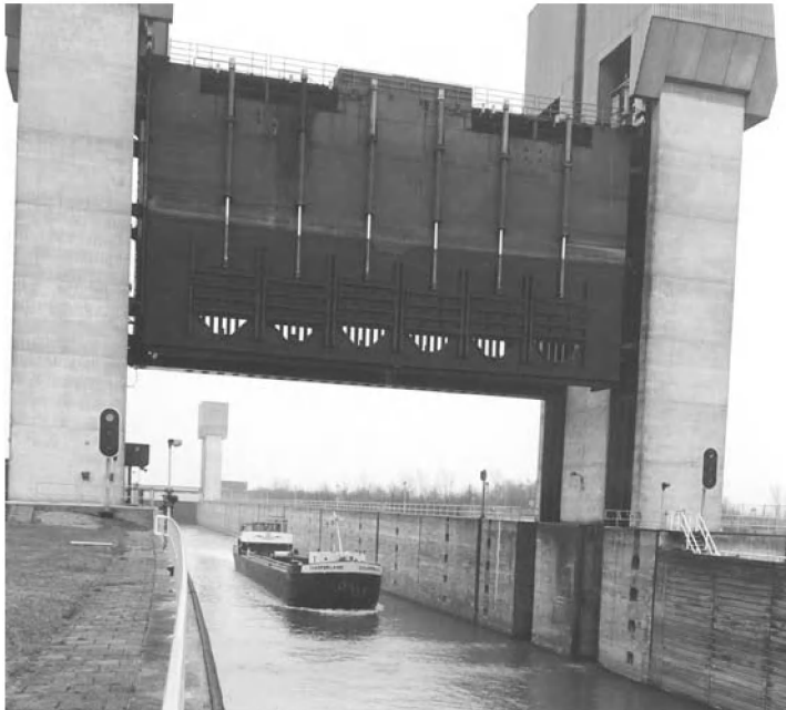
Photo 7.7 Lift gate at Prins Bernardsluis in Tiel
