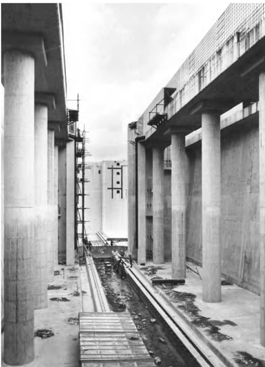
Photo 8.4 Gate chamber of rolling gate of the marine lock in Terneuzen
