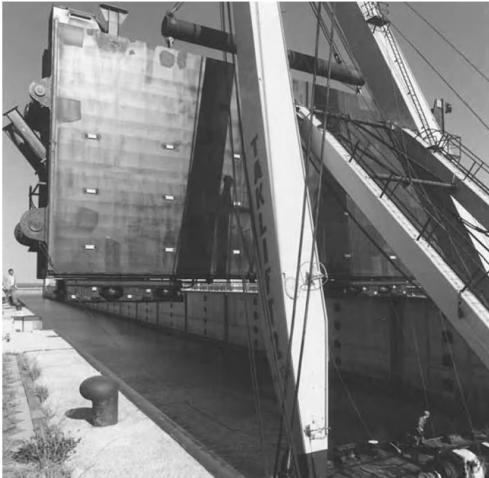
Photo 7.5 Rolling gate at Krammersluizen during installation (1985)
