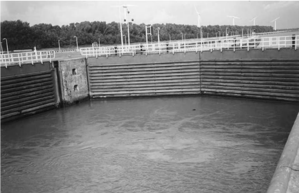
Photo 6.5 Flow pattern during filling by means of gate openings of the push-tow locks in the Volkerak
