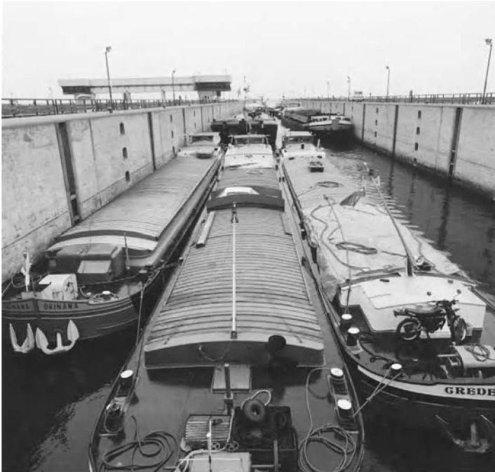
Photo 4.2 Push-tow navigation locks in the Kramer
