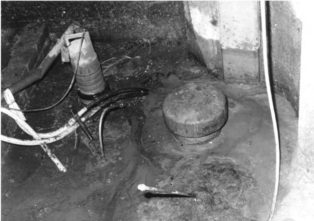
Photo 7.8 Bottom pivot of the mitre gates at Middensluis IJmuiden
