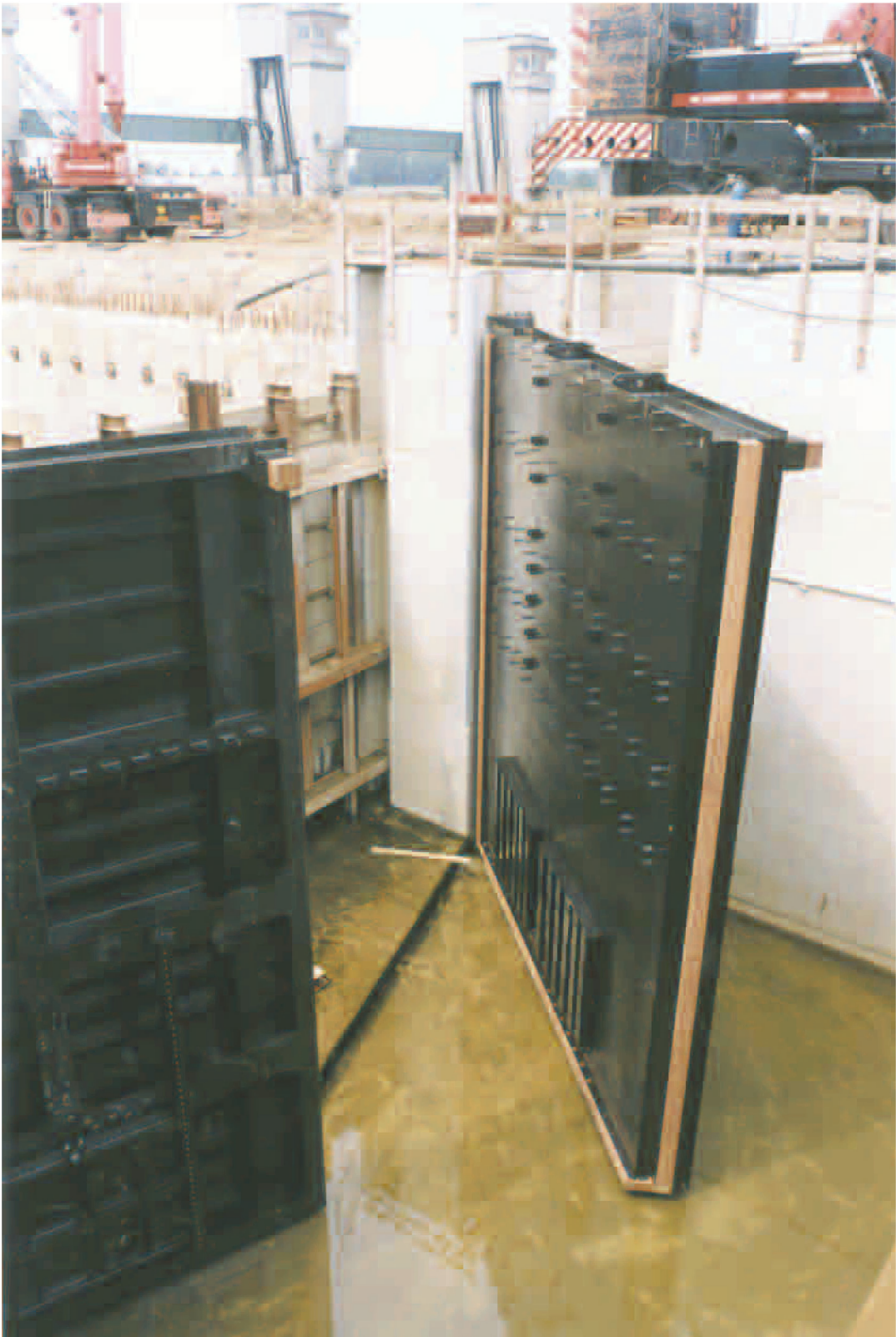
Photo 7.1 Mitre Gates at Tweede Sluis Lith during installation (1998)
