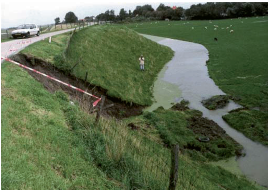
Figure 2-11 Example of sliding of the inner slope.
