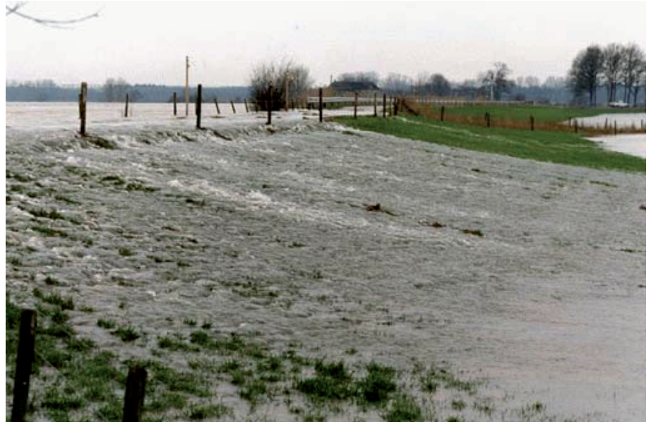
Figure 2-7 Flooding due to a dike overflow
