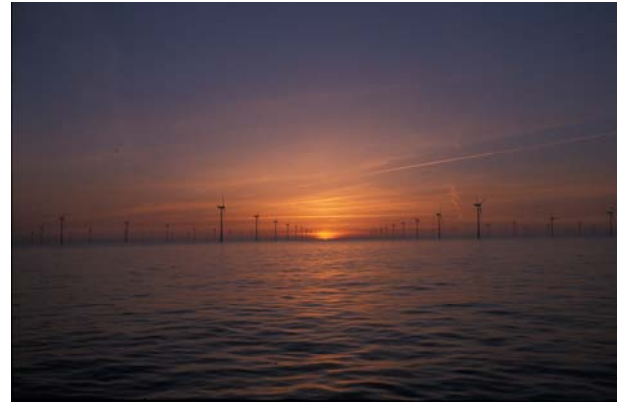
Photo 3. Horns Rev offshore wind farm.
