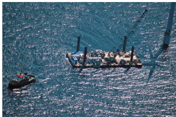
Photo 6. Horns Rev offshore wind farm under construction.
