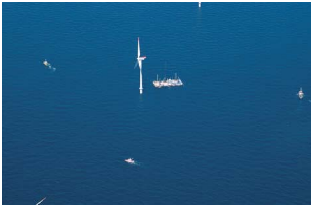
Photo 2. Horns Rev offshore wind farm under construction.
