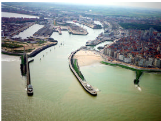
Fig. 1. Oostende harbour, present situation.
