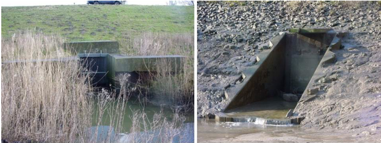
Figure 42 - Outlet entrance (on the left) and exit (on the right) in Lippebroek (Patrimoniumdatabank W&Z)
