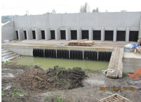
Figure 51 - Inlet and outlet culvert configuration on the river side (construction phase) (Patrimoniumdatabank W&Z)
