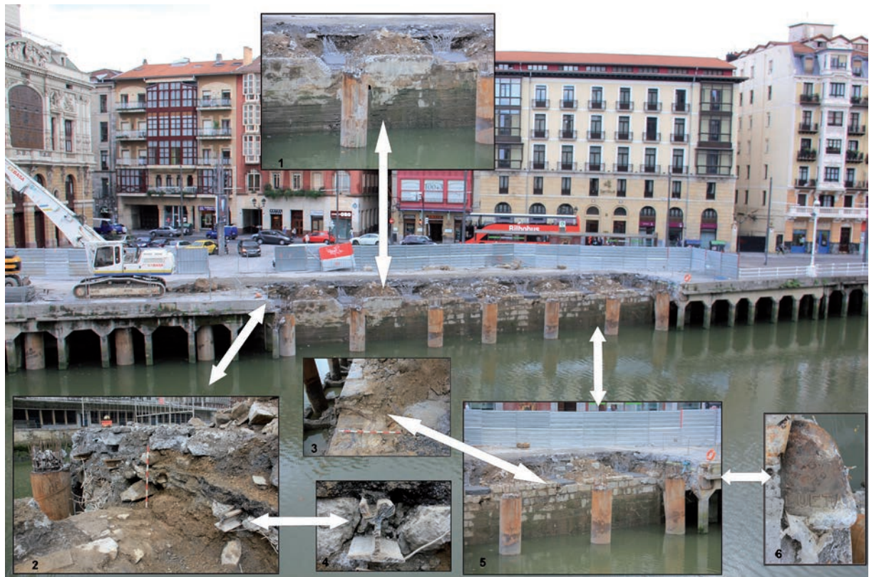
Figure 4. Frontwall of the Arriaga dock being repaired. 1) detail of the staircase being blocked once the platform was built; steps are visible; 2) detail of the rails, platform built in 1927 and the 1890 frontwall with the top of the staircase blocked; 3) detail of the mooring ring inside the frontwall; 4) Phoenix rail; 5) detail of the frontwall where the mooring ring is; 6) bollard found in situ (Photo J. M. Matés Luque).
