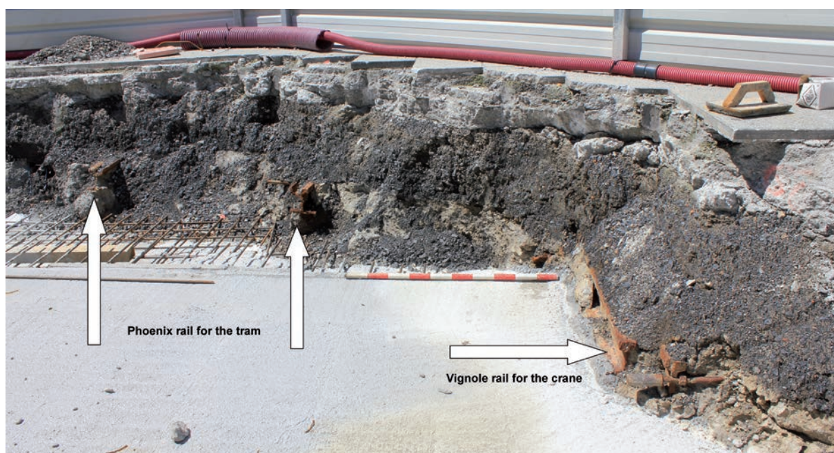
Figure 3. Detail of the rails recorded. The union of Vignole type for the cranes next to the riverbank and the Phoenix for the trams is common in Bilbao (Photo J. M. Matés Luque).
