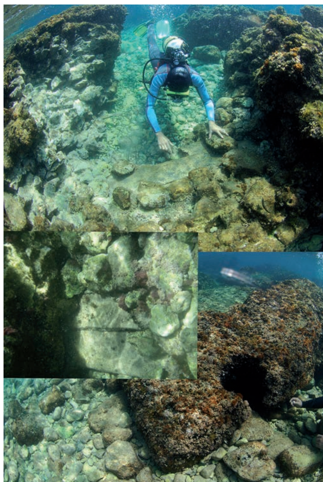
Figure 5. Otranto (Lecce, Italy). Ancient pier. Vertical hole (diameter 30 cm), impression in the concrete of the original internal post/pile ( destina ) and the timber board shuttering identified as the formwork bottom.
