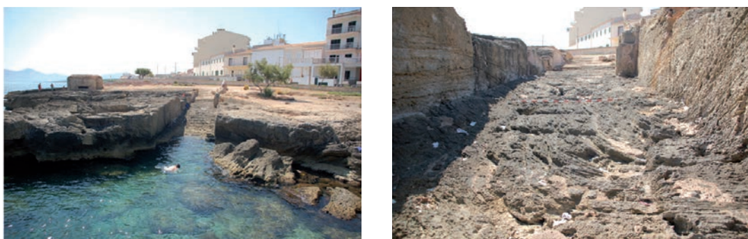
Figure 3. a) General view of the slipway from the sea; b) View up the slipway.
