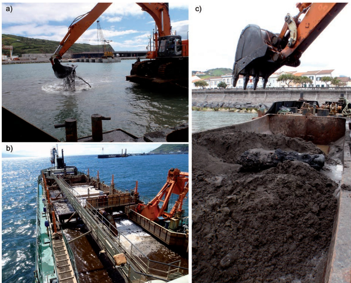
Figure 5. a) Dredging operations by a front shovel dredge b) Dredging operations by a trailing suction dredge in the area outside the harbor; c) a cannon, when discovered in BH-003 area during the archaeological monitoring of the shovel dredging. In the case of the suction dredger, archaeological monitoring was totally ineffective.
