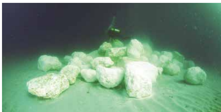
Fig. 1 – Artificial reefs made of limestone boulders to restore the rocky coral substrates, offsetting the impact of marine works to restore the sand along the beaches of the Miami county coastline in Florida, USA. © K. KILFOILE. ■
