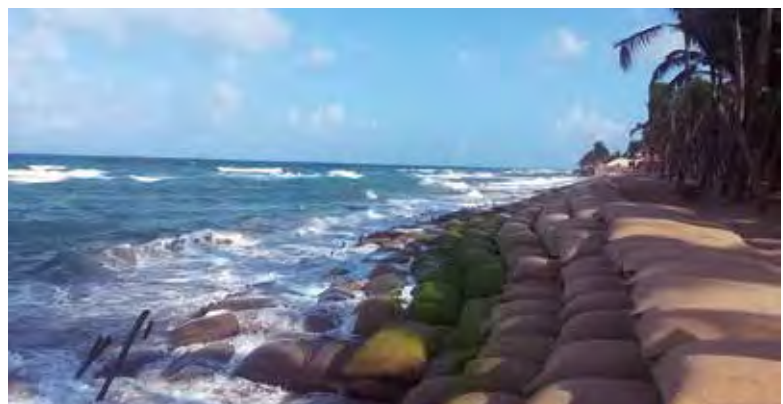
Fig. 1 – The city of Hoi-An in central Vietnam is included on the UNESCO World Heritage List. It used to be a prosperous city, thriving on maritime trade but its activity declined as its river silted up. Today, its beaches are subject to extreme erosion, requiring emergency but sustainable measures and therefore close understanding of the processes at work and predictive models. © R. ALMAR. ■
