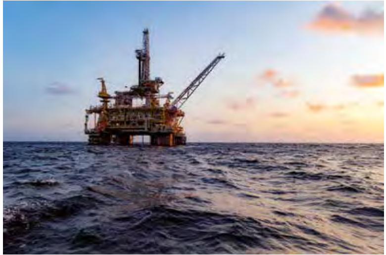
Fig. 2 – Full view of the Tension Leg Platform, Moho Nord Project, Total subsidiary E&P Congo. © D. MALFERE / TOTAL. ■
