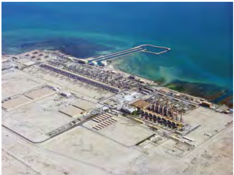
Seawater desalination plant in Doha, Qatar (2015). Source: tpe103eau.wordpress.com . ■
