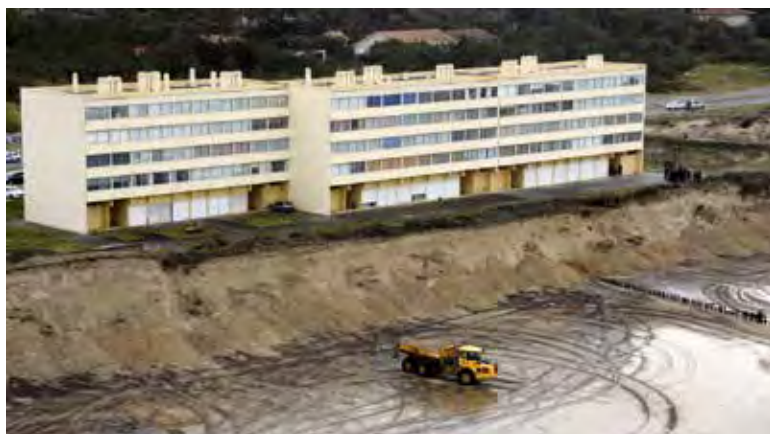
Fig. 1 – Built 200 m from the shore in the 1960s, the 'Le Signal' residential block at Soulac-sur-Mer was threatened by erosion and evacuated in January 2014. Source: France 3 Aquitaine. ■
