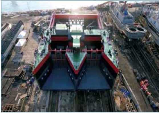
Construction of 300 kW floating pendulum WEC
