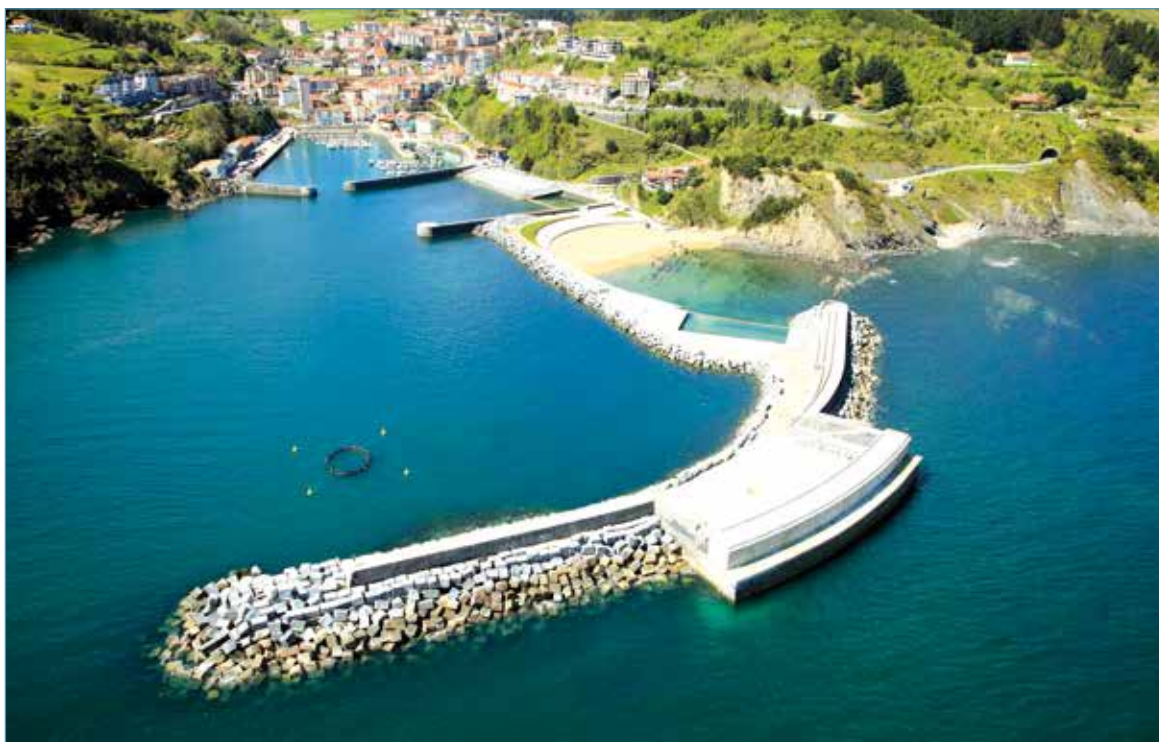
Mutriku wave power plant
