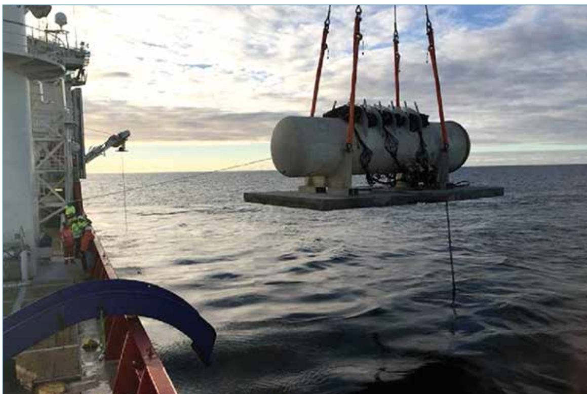
Deployment of the low voltage marine substation in the Sotenäs project
