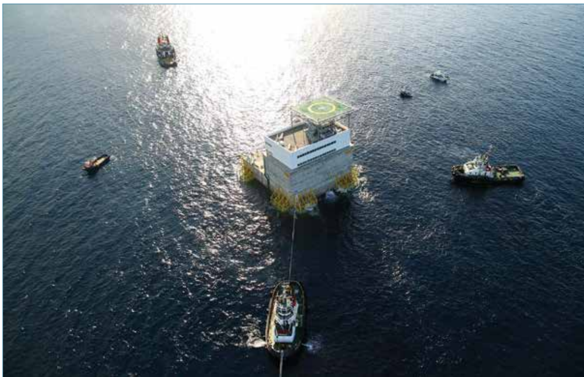
Installation of PLOCAN offshore platform
