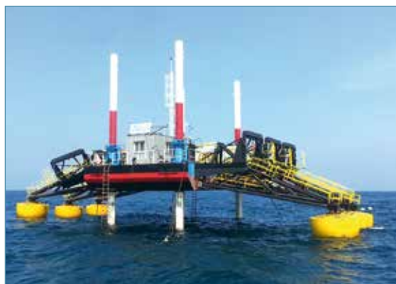
Heaving semi-sphere WEC with hinged arm
