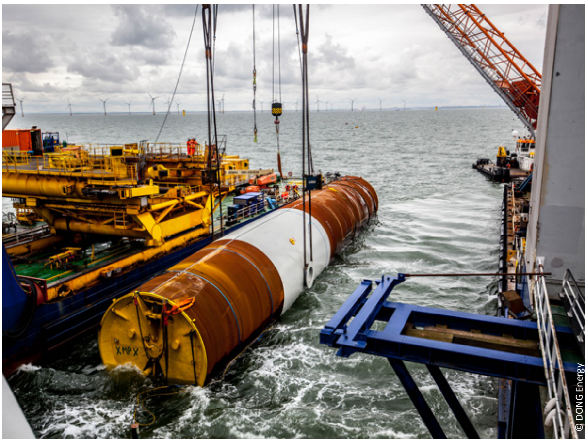
Monopile foundation installation
