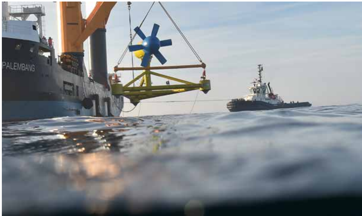
Sabella D10 tidal turbine deployed off Ushant Island
