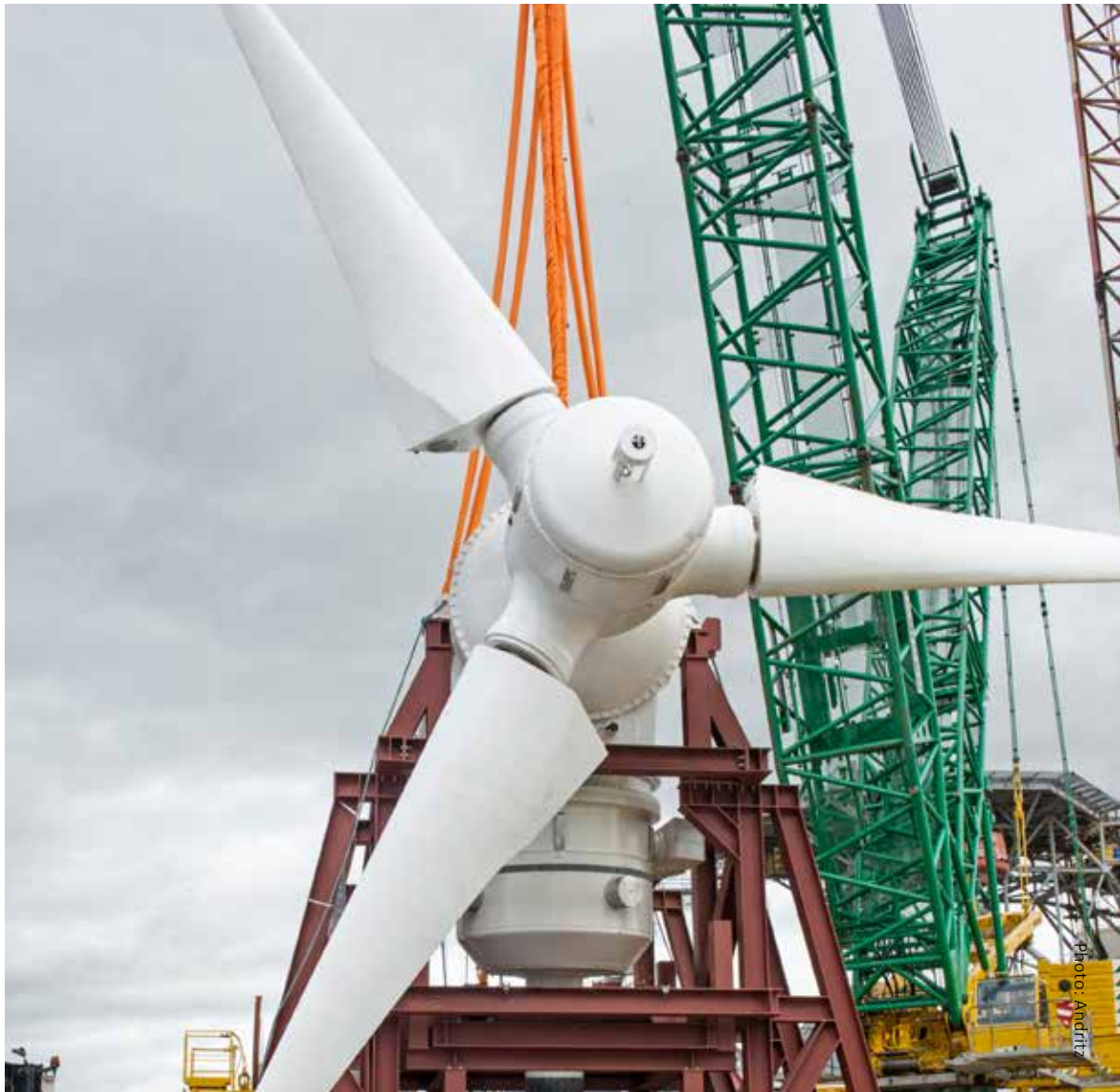
Andritz Hydro Hammerfest tidal turbine ready for deployment at the Meygen Project in Scotland
