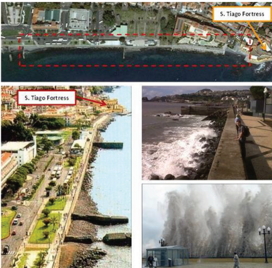
Figure 17: Waterfront of the east side of Funchal before intervention
