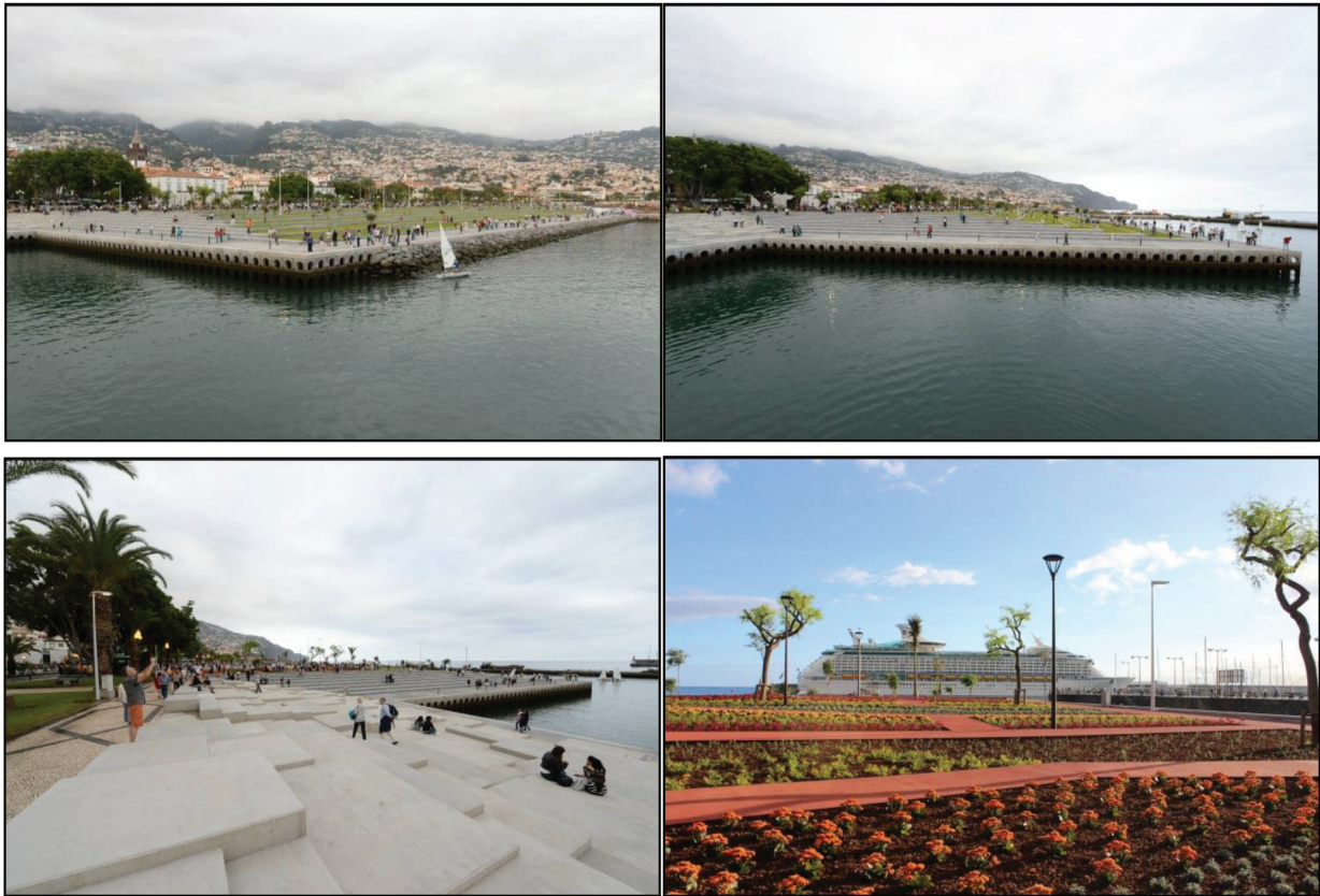
Figure 16: The inner dock and the garden (Source: Courtesy of the Autonomous Government of Madeira)
