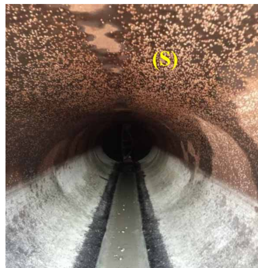
Figure 1 | Marine shells (s) in a feed water line of an MSF desalination plant on the Gulf coast.
