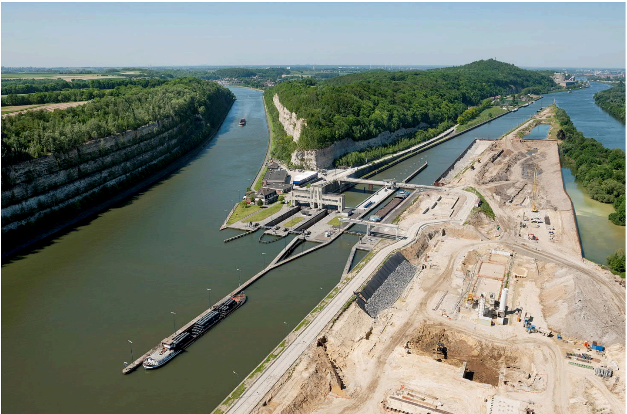
Fig.8: Overall view during excavations– © JL DERU/photo-daylight
