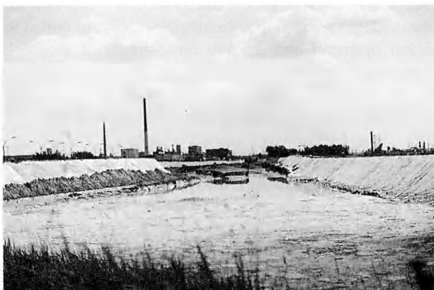
Fig. 71A — Sea-Scheldt dike. Slurry wall ditch.
