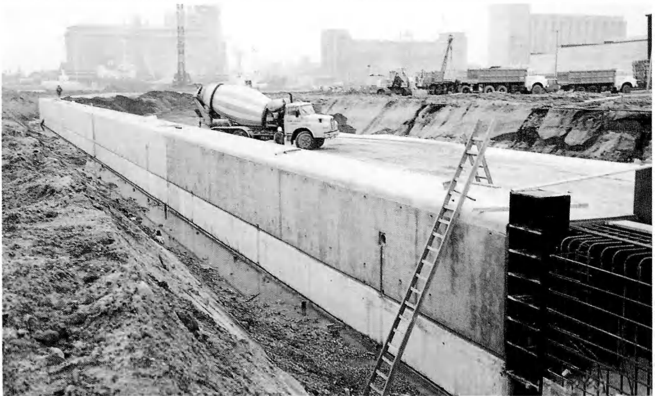
Fig. 56 — Quay wall section after being concreted.
