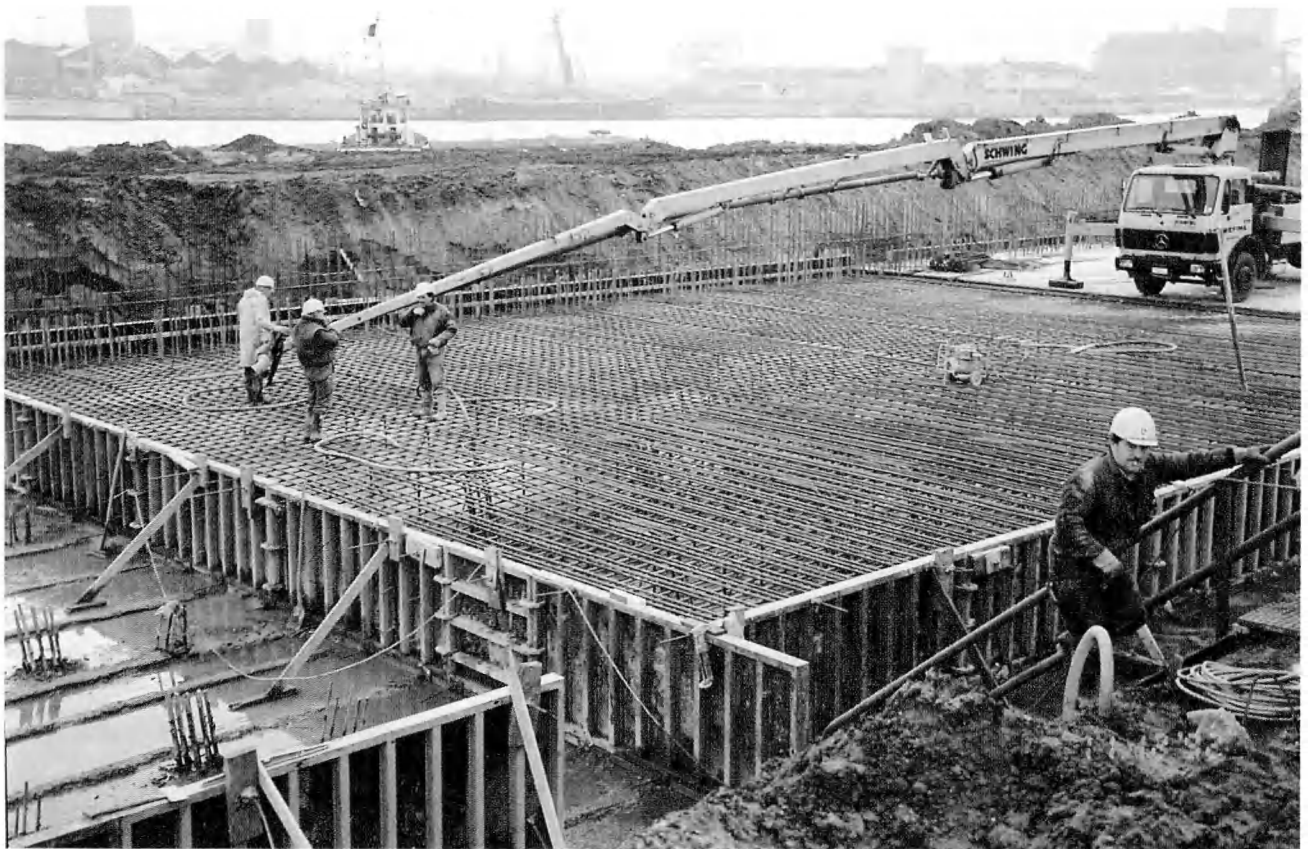
Fig. 55A — Reinforcement and shuttering of the top slab (standard section).
