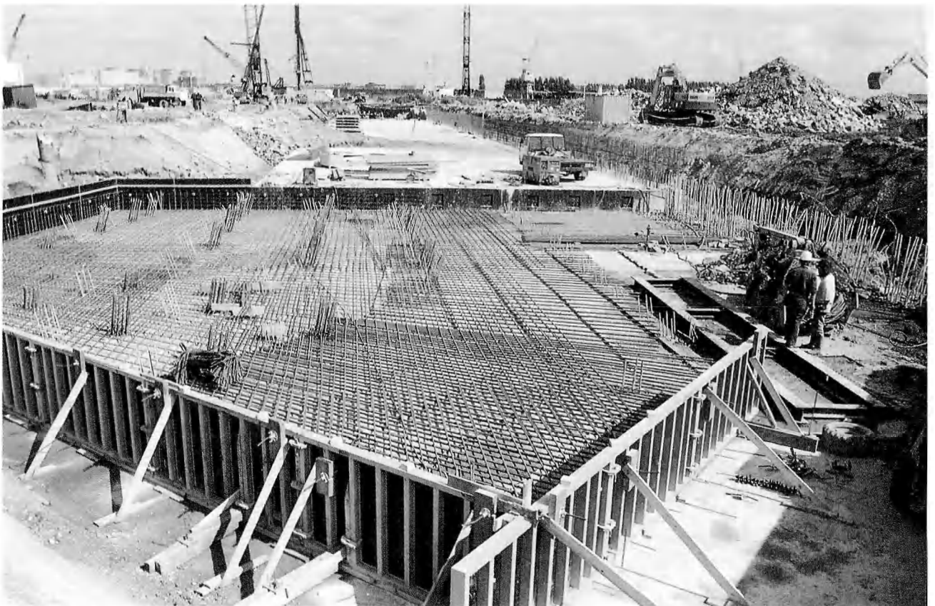
Fig. 55B — Reinforcement and shuttering of the top slab (corner section).
