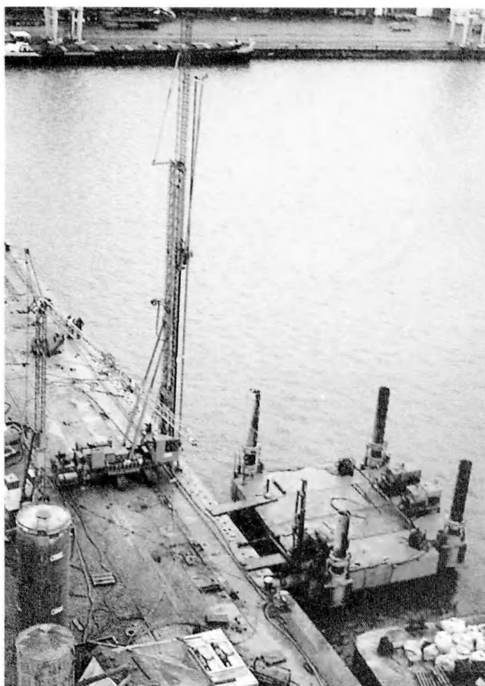
Fig. 95 — Very High Pressure grouting. Application.
