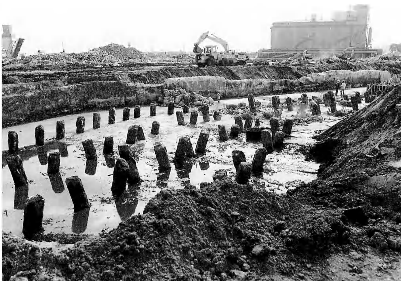
Fig. 51 — Pile heads after the excavation.
