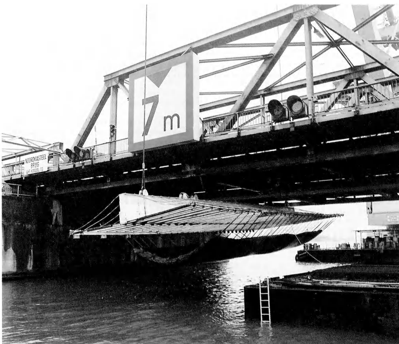
Fig. 74 — Placing of the fiberised open stone asphalt mats under the fixed bridge deck section.
