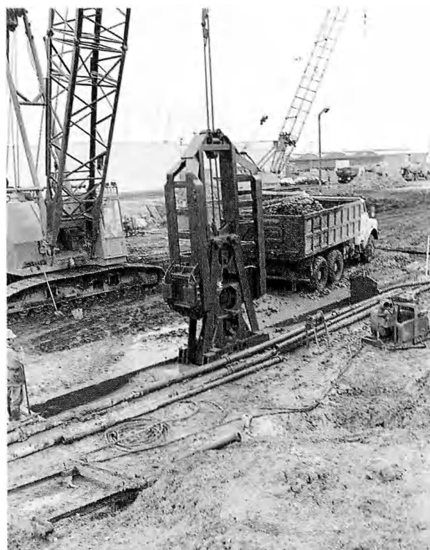
Fig. 41 — Slurry wall construction — Excavation of trench with a grabcrane between guide walls.
