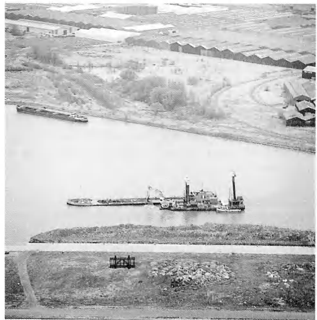
Fig. 69 — Dipper dredger "Zenne" while excavating the renovated quay wall (in the background the future site for the new shelter dock for lighters).
