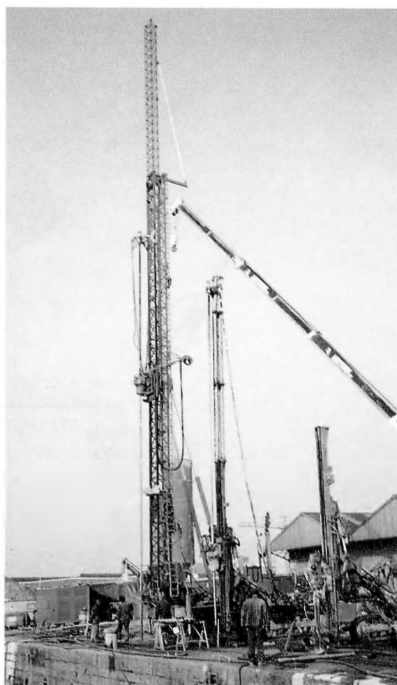
Fig. 95 — Very High Pressure grouting. Application.
