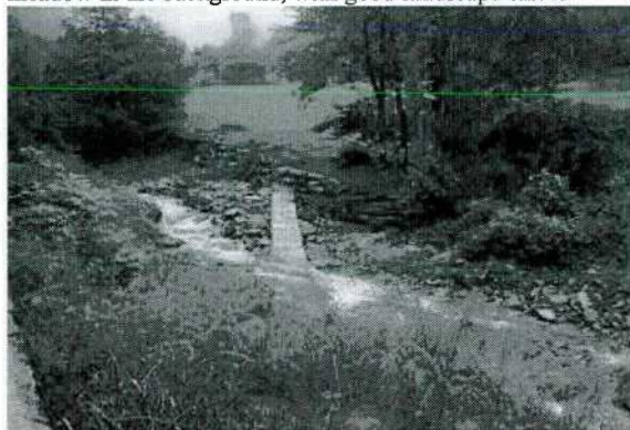
Figure 6.4: An interred penstock crosses the river and the meadow in the background, with good landscape effect
