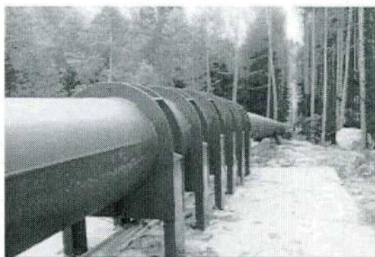
Figure 6.5: an uncovered anchoring block at 600 mm-diameter penstock without expansion joints.
