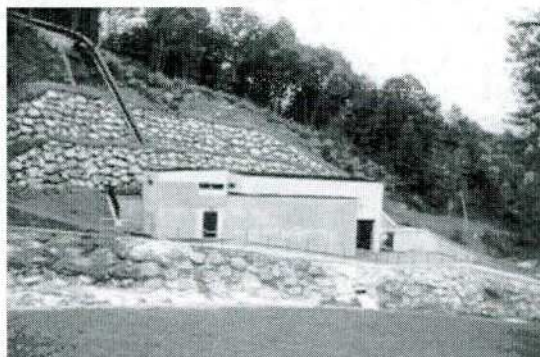
Figure 6.8: a combined intervention for slopes consolidation at a small hydropower plant.
