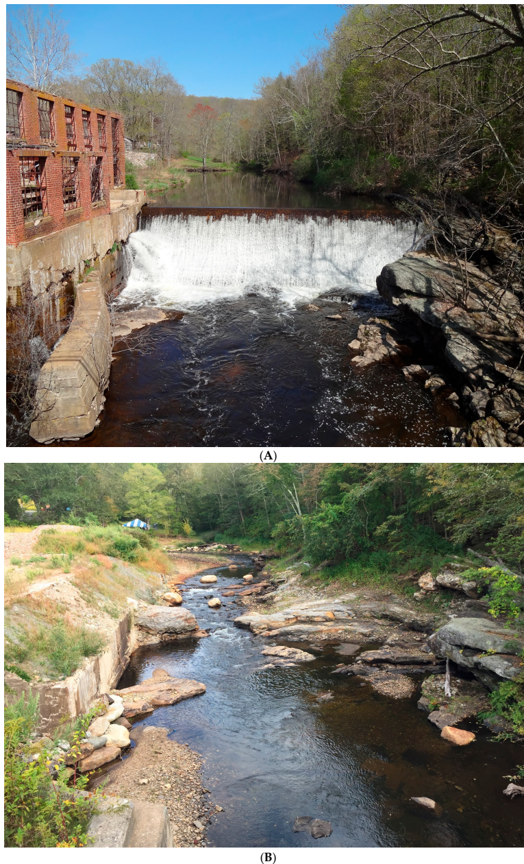
Figure 1. The Norton Mill Dam (A) was located on the Jeremy River in Colchester, CT. The 12-foot high dam served an adjacent paper mill until the mill closed in the 1960s. Removal of this dam (B) opened 17 miles of high quality, forested, ‘trout-stream’ habitat and will benefit Atlantic salmon ( Salmo salar ), sea-run brown trout ( Salmo trutta ), sea lamprey ( Petromyzon marinus ), American eel ( Anguilla rostrata ), and Eastern brook trout ( Salvelinus fontinalis ). In addition, the dam was a threat to public safety from both upstream flooding and downstream flooding resulting from its failure. A submerged broken gate opening at the dam was an ongoing danger to boaters and swimmers who could have been trapped and drowned. The leaking dam undermined the structure of the adjacent brick mill, which could have led to a catastrophic collapse of a portion of the mill into the river, aggravating water control, flooding, and increasing jeopardy to the natural resources. Catastrophic failure of the dam would likely have resulted in damage to the CT Rt. 149 bridge, which is about 75 feet downstream of the dam, and would most likely have resulted in the scouring, undermining, and collapse of the Papermill Road bridge about 500 feet upstream of the dam (R. O. Bennett, personal communication and photo credit).
