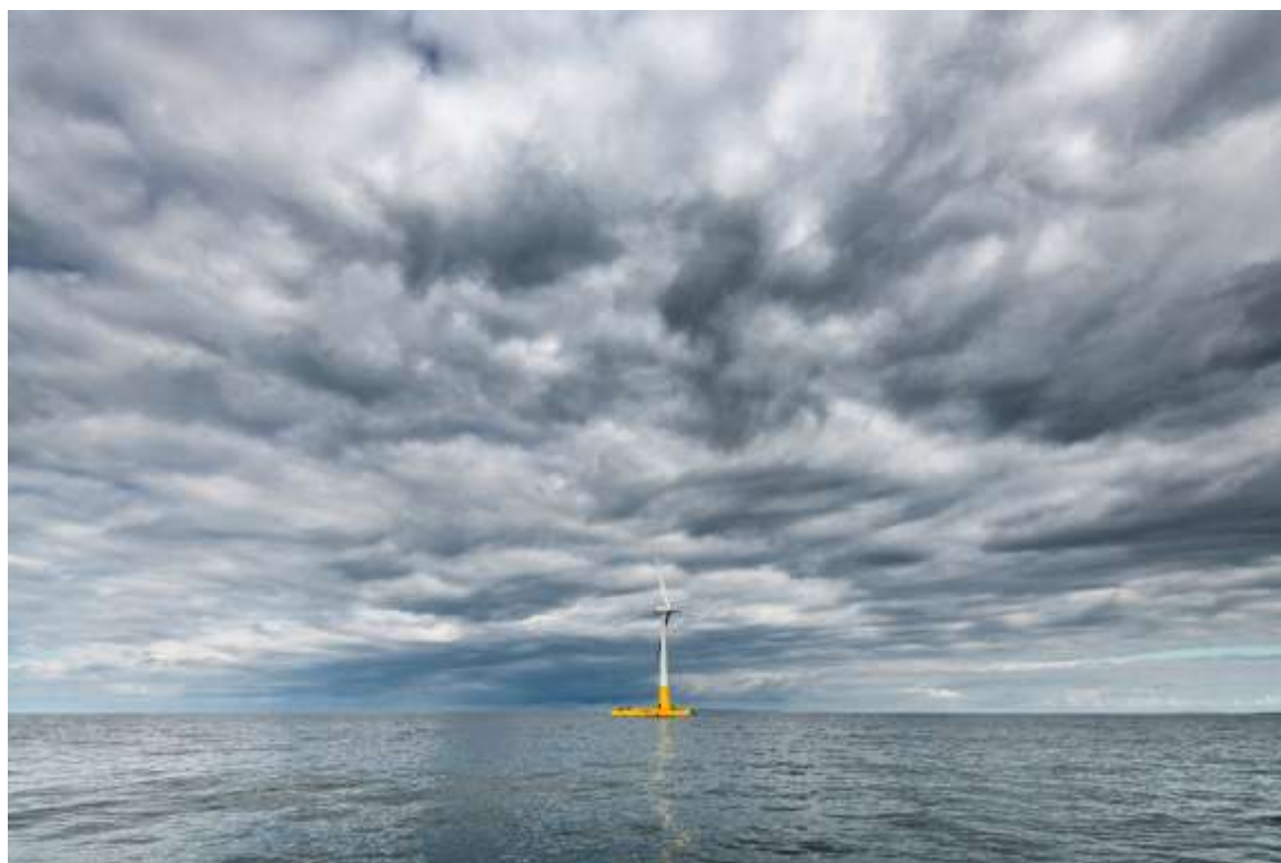
Figure 3. Floatgen Demonstrator, France, Picture credit: Ideol
