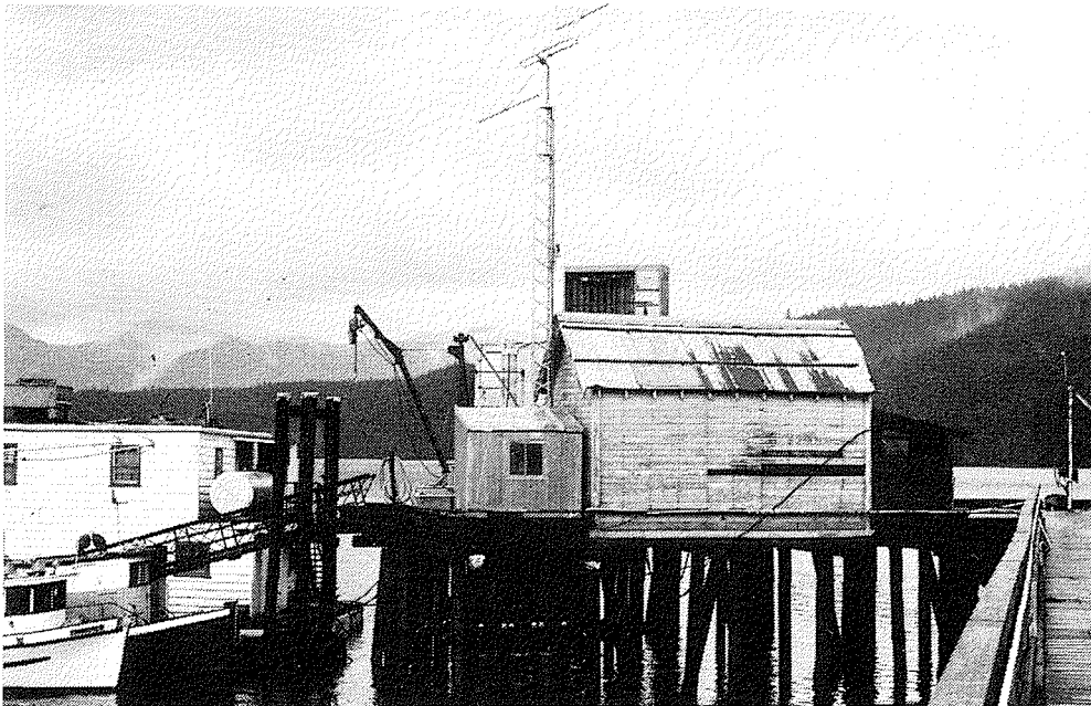
This Tsunami warning situation at Winter Harbour on the west coast of Vancouver Island uses the ionized trail left by meteorites as they strike Earth's atmosphere to flash messages from remote sights. The antenna is part of that meteor burst VHF radio transmission system.
